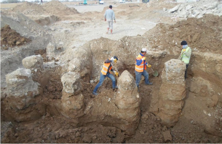
Fig. 2 Excavation around jet grout columns
