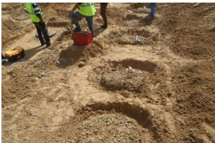
Fig. 4 Produced stone columns in test area
