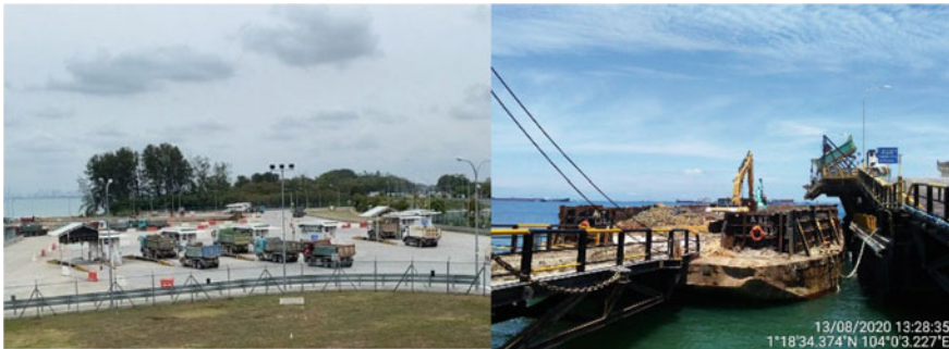
Fig. 1 (left) Excavated soil transported by dump trucks to the Staging Grounds, (right) Excavated soil loaded onto barges for transportation offshore
