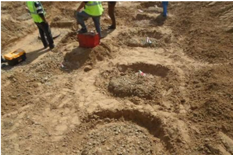
Fig. 4 Produced stone columns in test area
