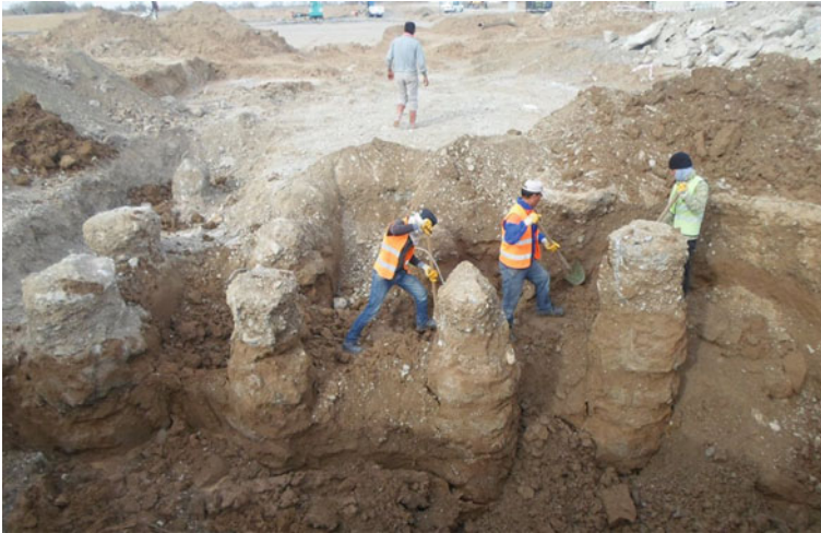
Fig. 2 Excavation around jet grout columns
