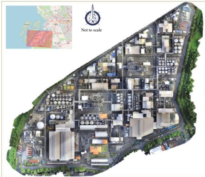
Fig. 1 Location of study in Heavy Industrial Area of Klang, Malaysia
