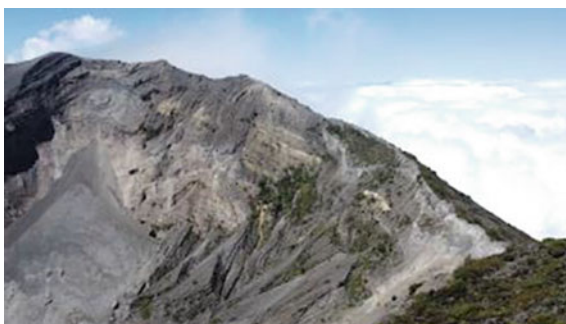
Fig. 25 Rockslides on the East crater wall
