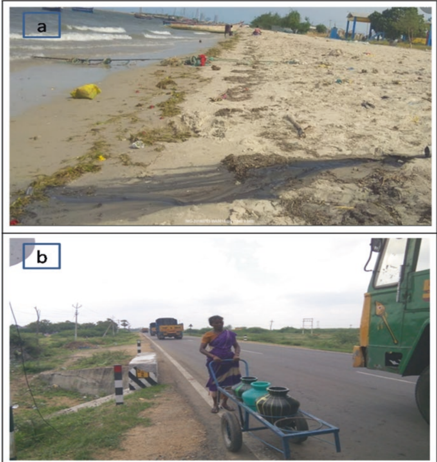
Fig. 26.11 (a) Sewage pipes are contaminating the Tuticorin coastal area. (b) Mela Arasadi people's search for freshwater
