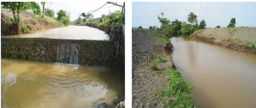
Fig. 28.2 Rainwater storage in deepened and widened drainage and CNB during kharif season 2016–2017
