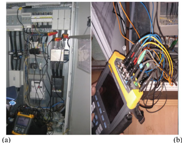
Fig. 15 PQ parameters measurement look on (a) whole cabinet and (b) instruments [12]
