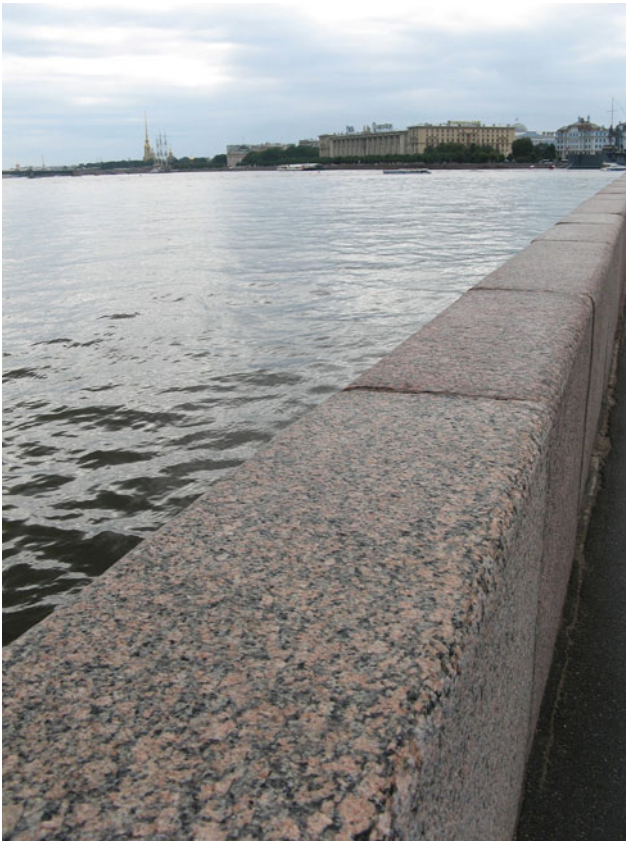
Fig. 12 Reconstruction of the Pirogovskaya embankment in 2010–2012: granites of the Ladozhskoye deposit
