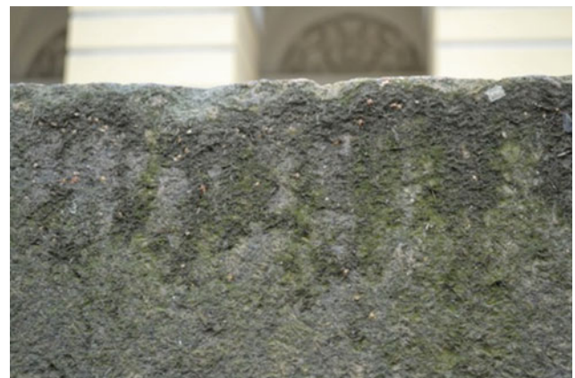
Fig. 13 Green algae-dominated biofilm associated with atmospheric pollution on the granite surface, St. Petersburg
