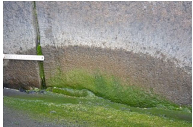
Fig. 12 Biofilm with dominance of green algae at the base of the granite facade of the Exchange building, St. Petersburg
