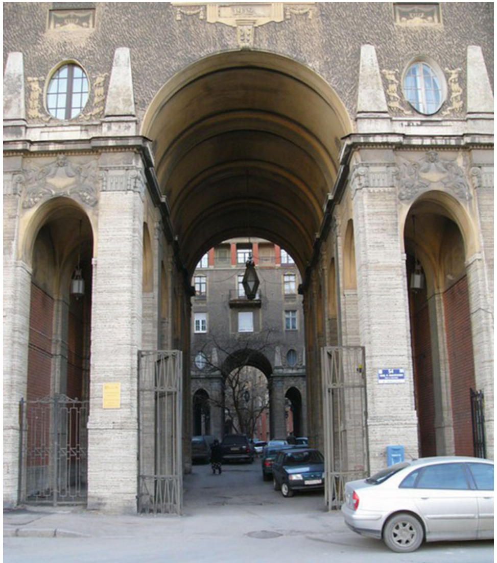
Fig. 7 Entrance group pylons
