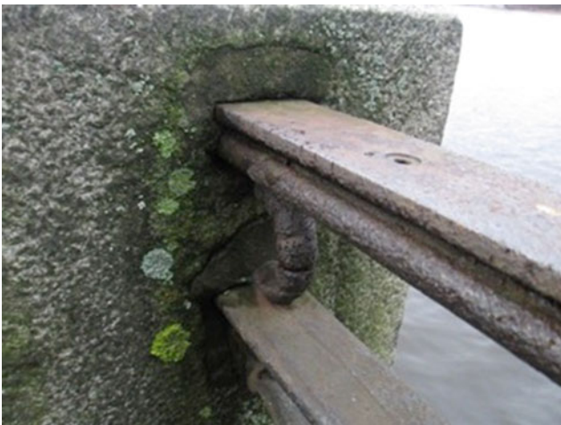
Fig. 24 Lichen fouling in the zone of contact between granite and cast-iron grating. Granite embankment. Vyborg
