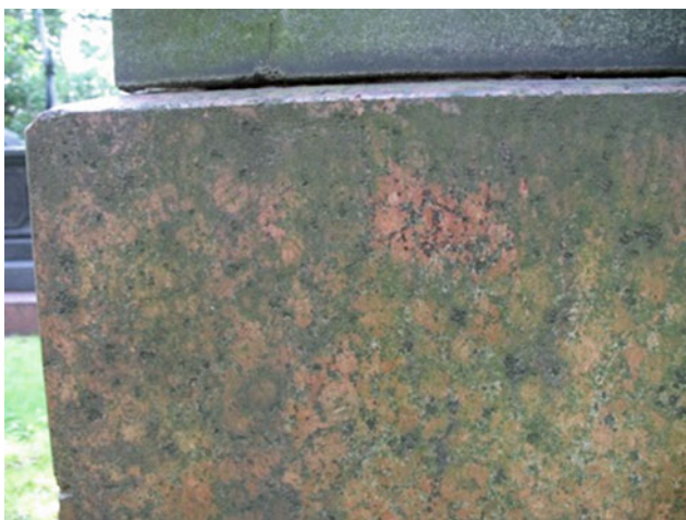
Fig. 10 Algae-dominated biofilm on a granite pedestal of a monument in the Museum Necropolis of the eighteenth century, St. Petersburg
