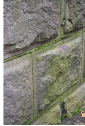
Fig. 11 Algae-dominated biofilm on the granite facade of a building in the Vyborg city
