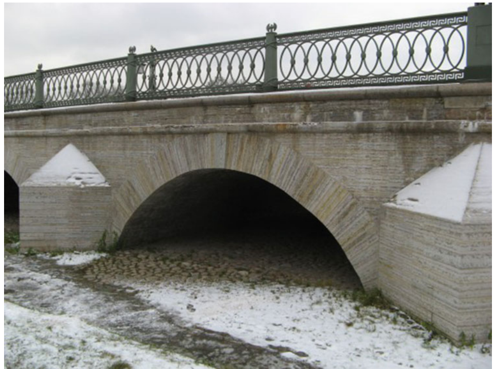
Fig. 10 Lining of trusses and abutments of the Ioannovsky Bridge
