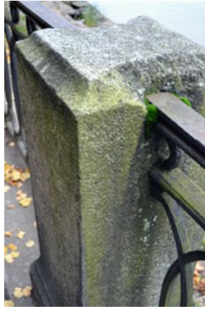
Fig. 9 Biofilm with algae dominance on the granite embankment in the Vyborg city
