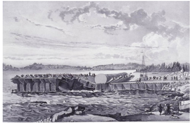
Fig. 8 Loading a column rod onto a barge (Montferrand 1836)
