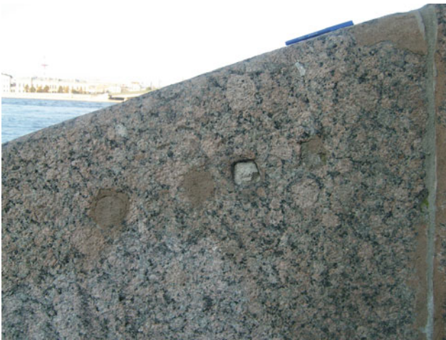
Fig. 29 Cementing of stone defects
