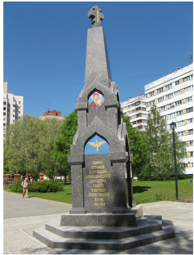
Fig. 4 Monument to the “Aviator Soldiers” in the Lev Matsievich Square between Bogatyrsky Avenue and Aerodromnaya Street, opened in 2019: rapakivi granites of the Vozrozhdenie deposit
