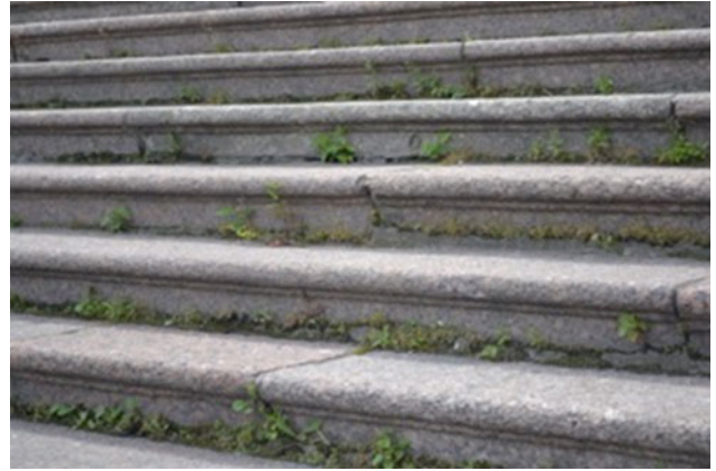
Fig. 25 Mosses and seed plants in the spaces between the granite steps. Exchange building. St. Petersburg
