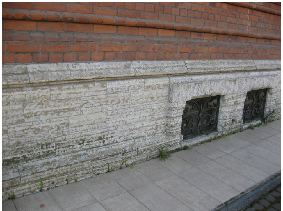
Fig. 2 Facing of the basement part of the facade
