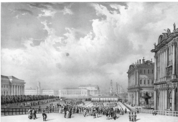
Fig. 10 Moving the finished column from the embankment to the overpass (Montferrand 1836)
