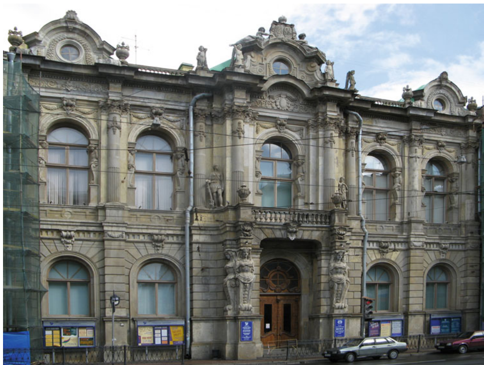
Fig. 1 General view of the front facade of building No. 42 on Liteyny Avenue
