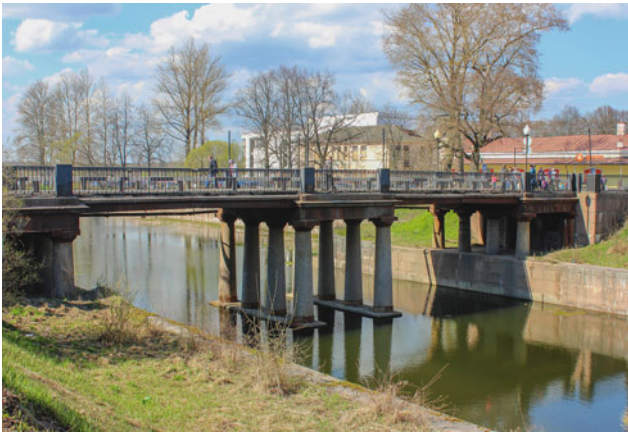
Fig. 18 Petrovsky Bridge in Shlisselburg
