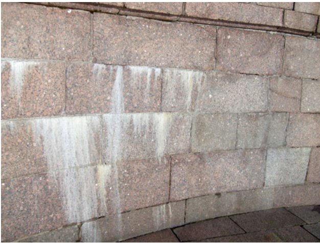
Fig. 30 Salt layer when cement dissolves
