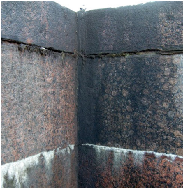
Fig. 18 Gray-black biofilm dominated by microscopic fungi on a granite embankment in St. Petersburg
