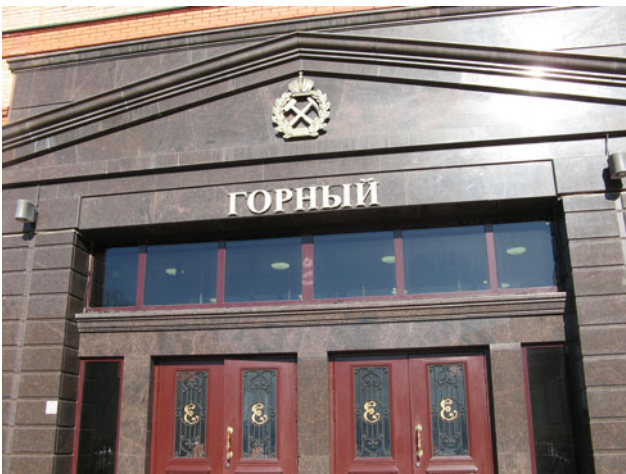
Fig. 6 Engineering building (academic building No. 3) of St. Petersburg Mining University, opened in 2015: in the photo, granosienites of the Ojararvi massif of deposits
