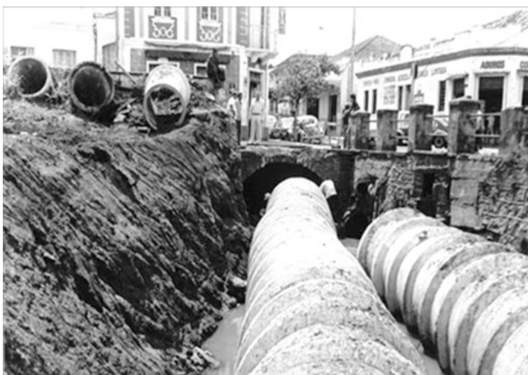
Fig. 9.4 Image Channelization of Gregório Stream, mid-twentieth century, main water body in the Gregório Basin, center of São Carlos city. (São Carlos Pro-Memory Foundation, undated)
