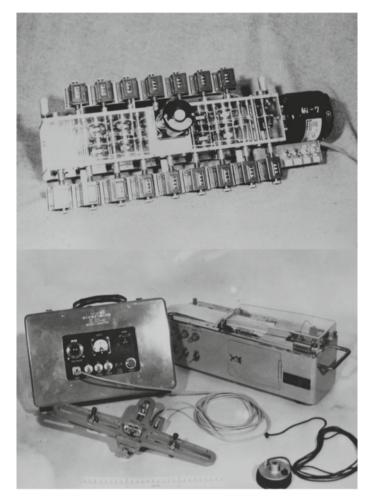
Fig. 3 Undulation measuring devices developed by Teru Hayashi
