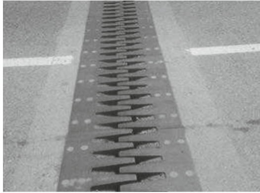
Fig. 1. Schematic diagram of highway bridge expansion joints
