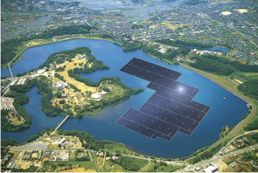
Fig. 8.3 Photovoltaic power plant floats on water at the reservoir of Yamakura Dam, Chiba Province, Japan. Source https://www.pv-magazine.com/2018/03/27/kyocera-jv-inaugurates-13-7-mw-floating-pv-plant-in-japan/
