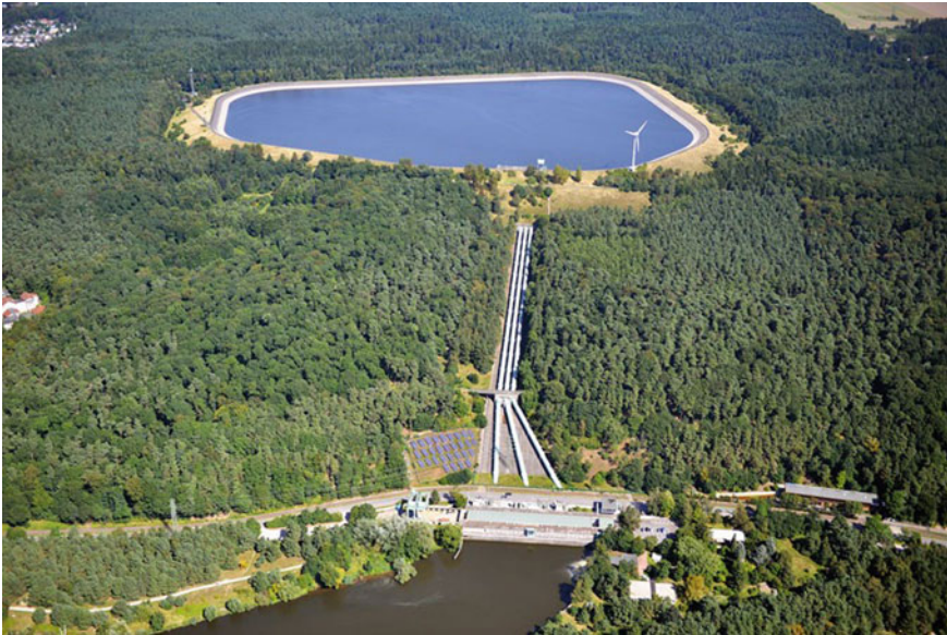
Fig. 8.2 Geesthacht pumped storage power plant, near Hamburg, has been operating since 1958. Source https://powerplants.vattenfall.com/geesthacht
