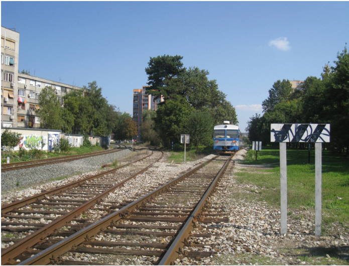
Fig. 9. Railway towards the Osijek eastern industrial zone – current situation.
