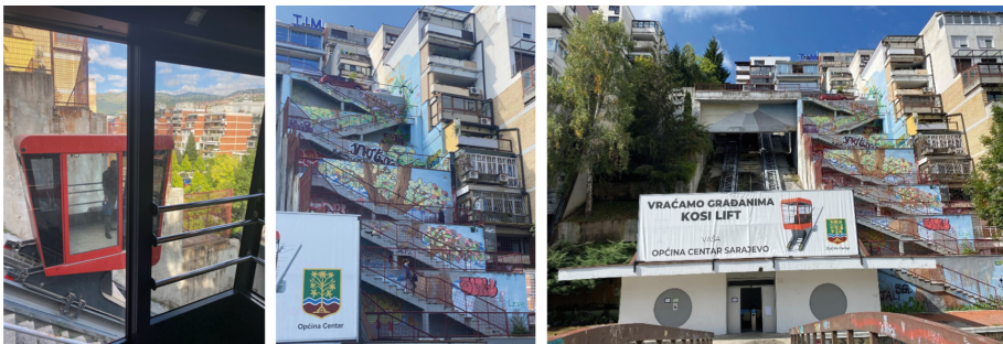
Fig. 3. The Exterior hillside elevator and supporting exterior stairs at the Ciglane residential complex illustrate a unique and technologically advanced feature for its time.
