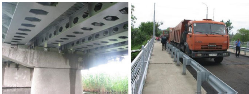
Fig. 13 Composite reinforced concrete bridge in Barvenkovo (author's photo)
