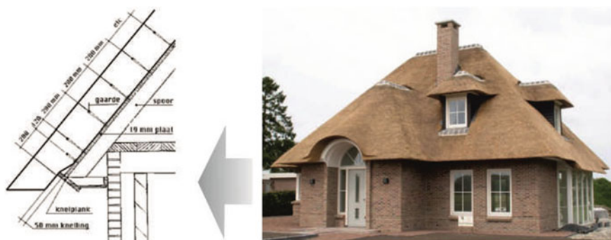
Fig. 1 “Dutch” method of covering roofs with reeds. Source [17]
