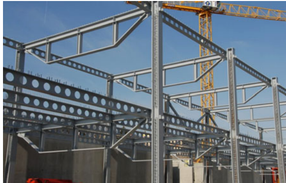
Fig. 1 Combined steel trusses with I-beam stiffness beam [4]
