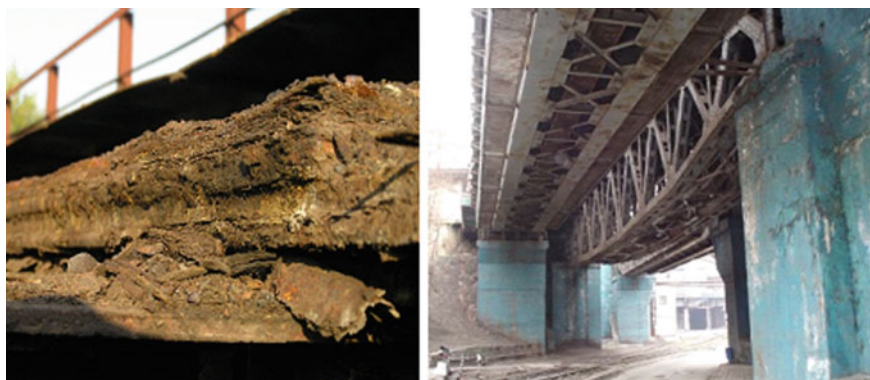
Fig. 3 Monitoring of bridge structures
