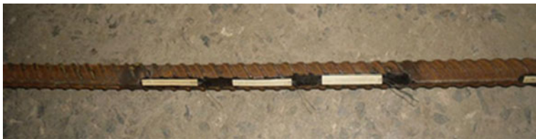
Fig. 5 General views of the resistance strain gauges in the test specimen—concrete beam BSR
