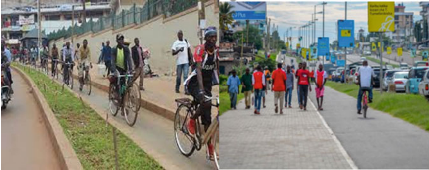
Fig. 19.3 Separated cycle lanes and pedestrian walkways
