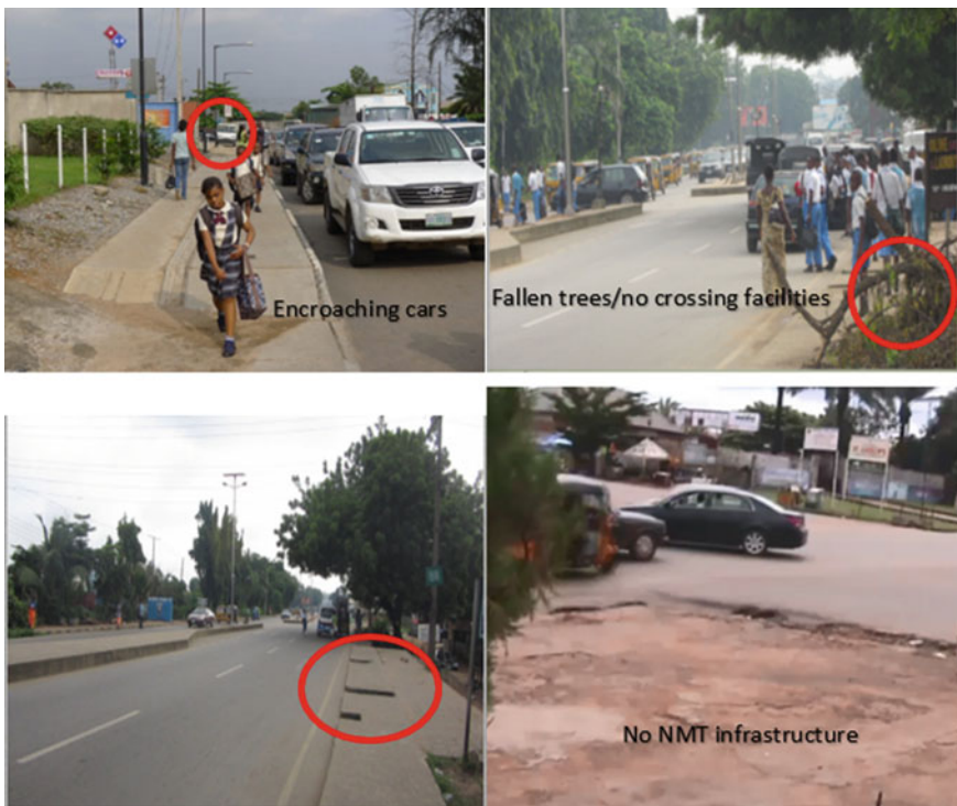
Fig. 19.2 State of some NMT infrastructures in some African cities
