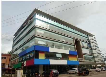
Fig. 2. Exterior of the commercial building.
