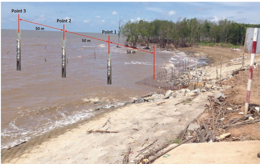
Fig. 3 Study sections and positions of wave measure equipment installation
