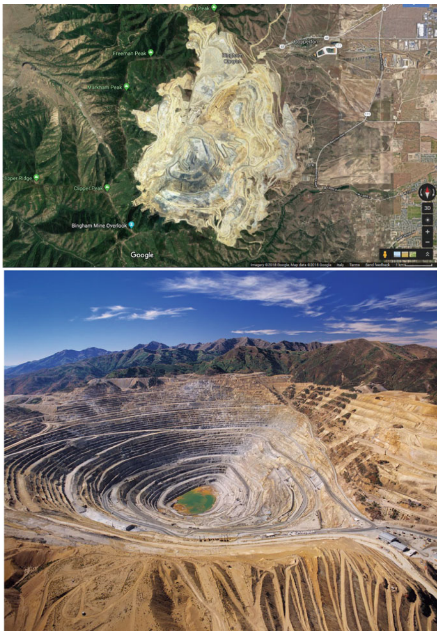
Fig. 8 Google Earth view of the Bingham mine open pit, Utah. The pit of the copper mine is possibly the largest hole created by man on Earth's surface
