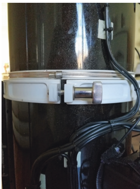
Fig. 7.5 Large cable bundle secured by the use of Pads and tie wraps
