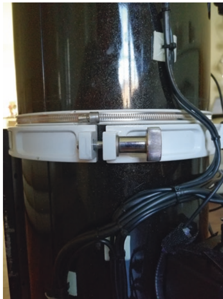
Fig. 8.55 Cable run fixed to the telescope tube
