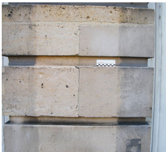
Fig. 19.2 Cleaning results on sample surfaces with different natural stone substrates. [Photo: Remmers]
