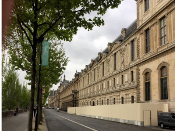
Fig. 19.7 First section of the Louvre façade cleaned with “Clean Galena” [Photo: Remmers]
