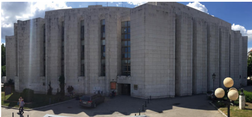
Fig. 17.2 Northwest-facing façade with the side entrance to the Serbian National Theatre building, before cleaning and protection works in 2021 (authors' photo)
