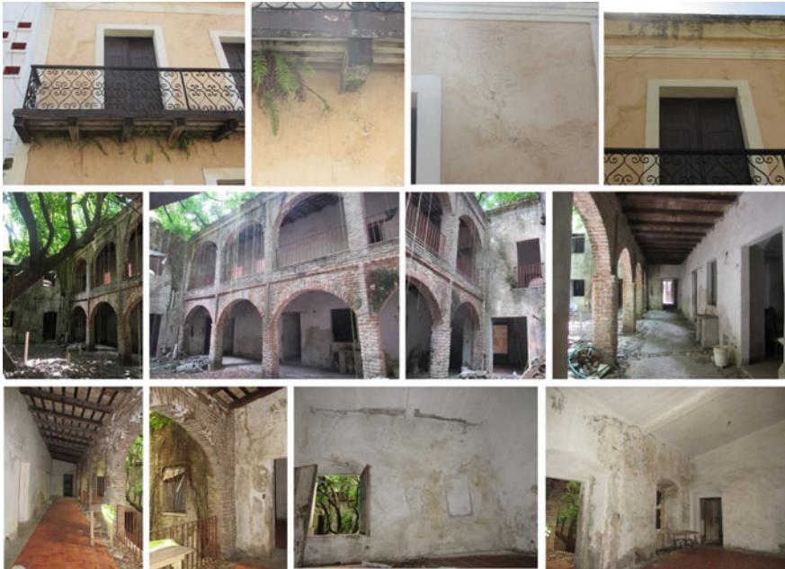
Fig. 7.3 Current building condition
