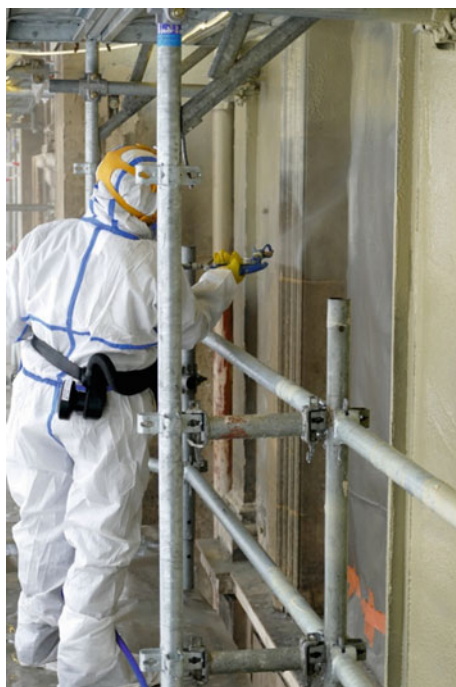
Fig. 19.11 Application of the cleaning compress at the Musée Carnavalet, Paris [Photo: H. Chevalier]
