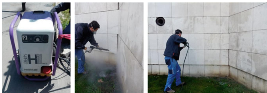
Fig. 17.5 Hot box machine (left photo) and hot box cleaning process (middle and right photos)
