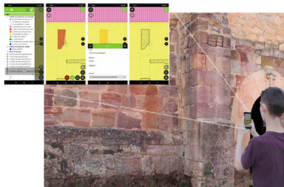
Fig. 6.8 Capture of on-site data through the QField application
