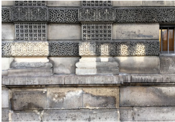
Fig. 19.3 Cleaning sample areas at the Louvre, Paris [Photo: Tollis]
