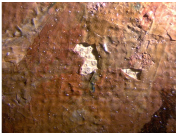
Fig. 10.4 Example of a paint layer flaking. Photograph shot through the microscope
