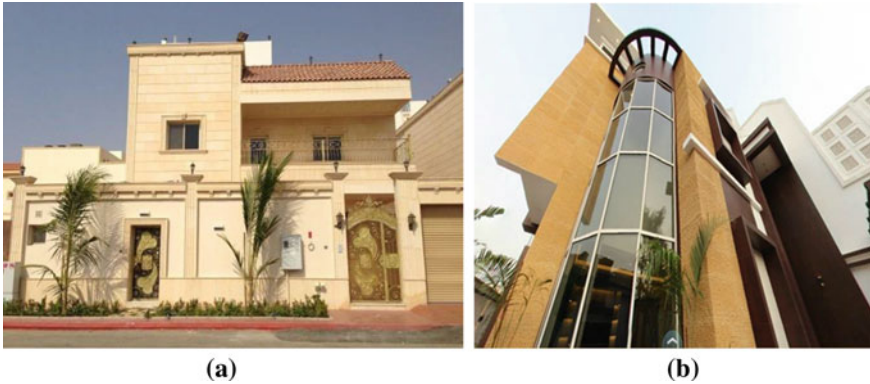
Fig. 10 Buildings in Al-Basateen (Photos taken by the author)
