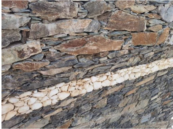
Fig. 6 Close up picture of the bricks on the castles. Source Authors
