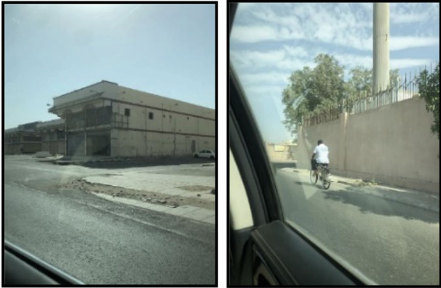
Fig. 15 Poor and low maintained pathways. Source Authors
