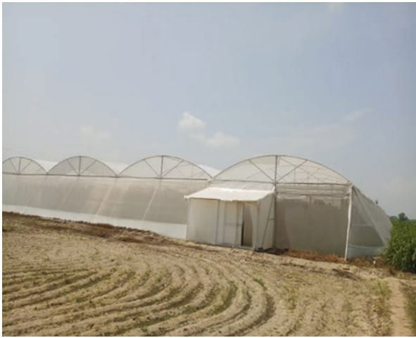
Fig. 16.3 Dome Shape Net House
