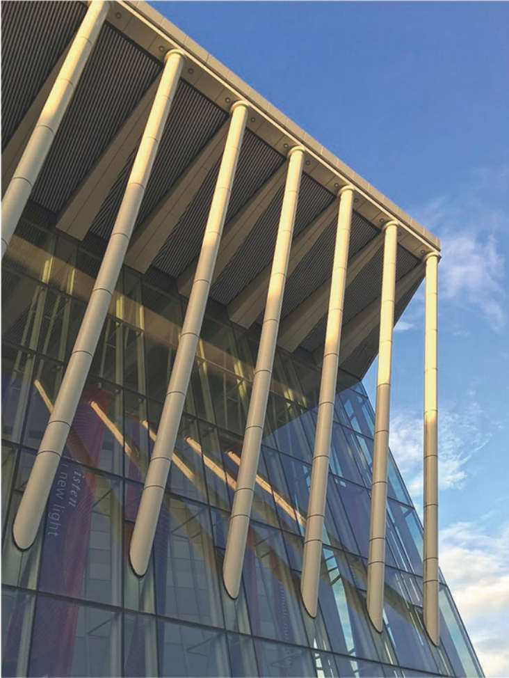
Fig. 22 Glazed façade of the Yong Siew Toh Conservatory at the National University of Singapore, Singapore. (Image credit and source: Joshua Rommel Hayag Vargas, https://commons.wikimedia.org/wiki/File:YST_Conservatory,_National_University_of_Singapore,_February_2020.jpg )
