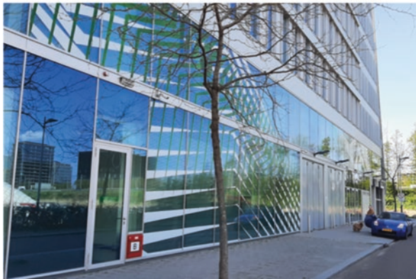
(b) The façade with smart glazing to control heat losses in winter and heat gain in summer months
