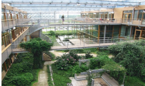
(b) Large green space covering most the interior under glass roof to cool and save energy.
