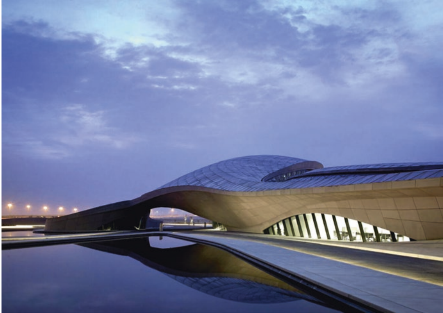
Fig. 12 General view of the envelope and roof of BEEAH Headquarters' net-zero and smart building at night. (Image credit and source: Hufton Crow, https://www.zahadidarchitect.com )
