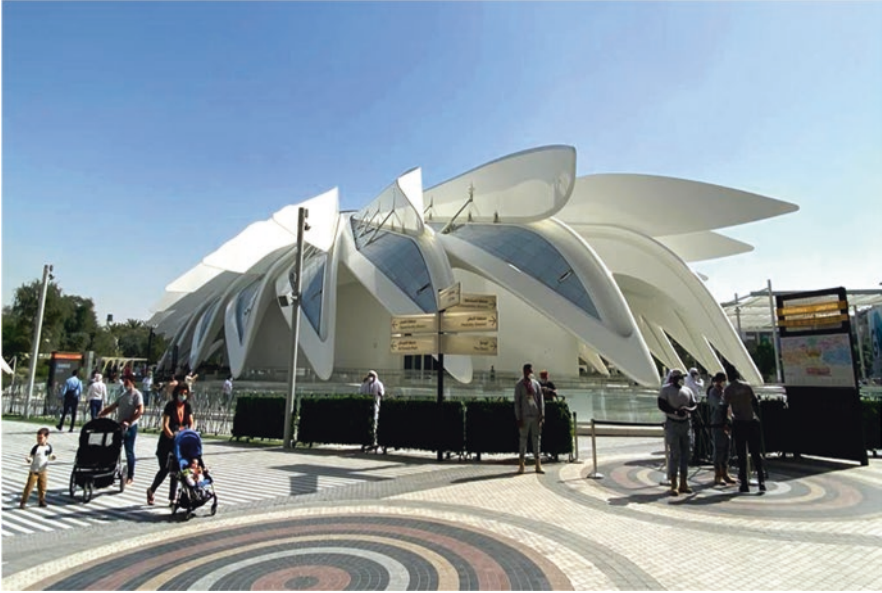
Fig. 16 The iconic UAE Pavilion with 28 floating wings integrating solar PV panels, EXPO 2020 Dubai. (Image credit and source: Mohsen Aboulnaga and Amina El-Haggan)
