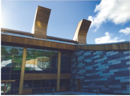
(a) Entrance to GSK Laboratory and its façades with efficient glass and cladding to save energy.
