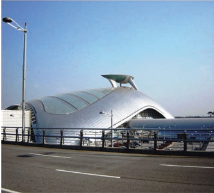
(a) The terminal's façade fixed with smart glass by Saint Gobain to protect it from sun radiation.
