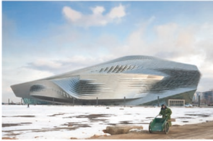
(a) Dalian Conference Center's external façade acts as a screen light penetration
