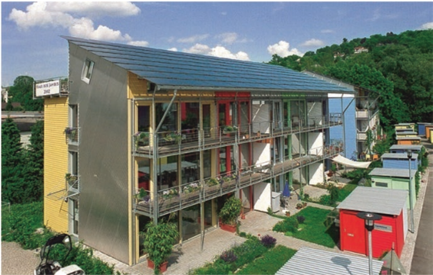
Fig. 47 View of the 91 solar PV array covering the tilted roof of the net-zero houses. (Image credit and source: Andrewglaser, https://commons.m.wikimedia.org/wiki/File:SoSie%2BSoSchiff_Ansicht.jpg#mw-jump-to-license )
