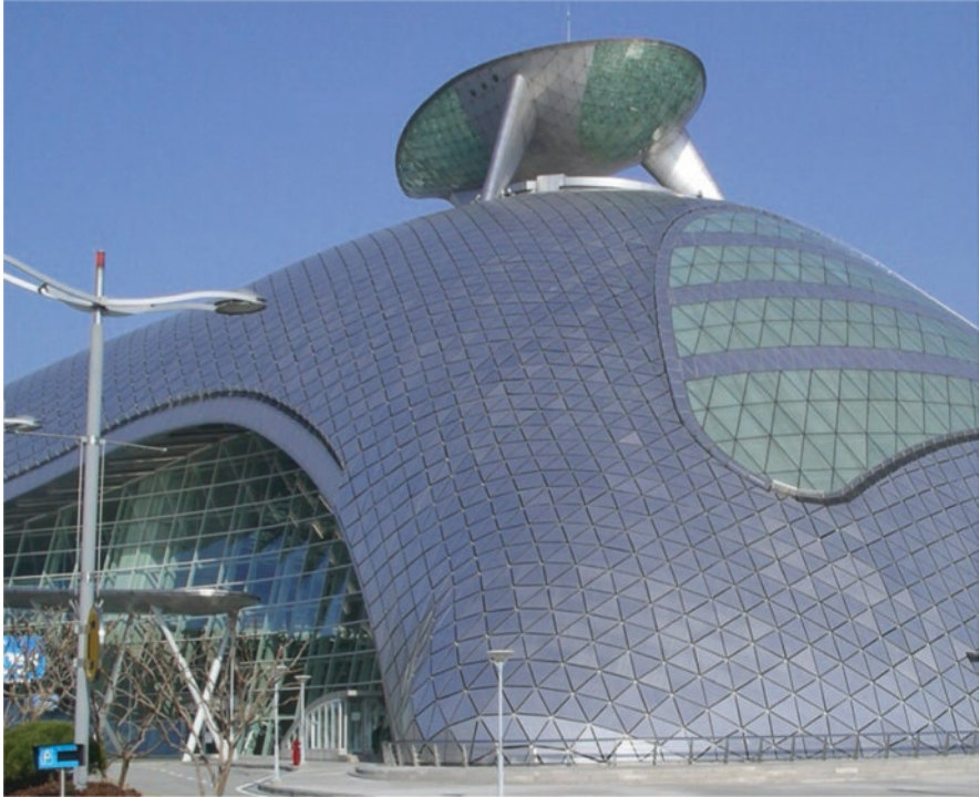
Fig. 28 Incheon-Seoul Airport Terminal envelope engulfs cells that contain titanium oxide coats with a photoelectric dye for generating electrical power for lighting and temperature control. (Image credit and source: Mohsen Aboulnaga, 2015)
