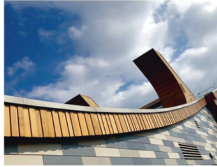
(b) Close up of the roof line with chimneys on the rooftop to promote natural ventilation and clean air
