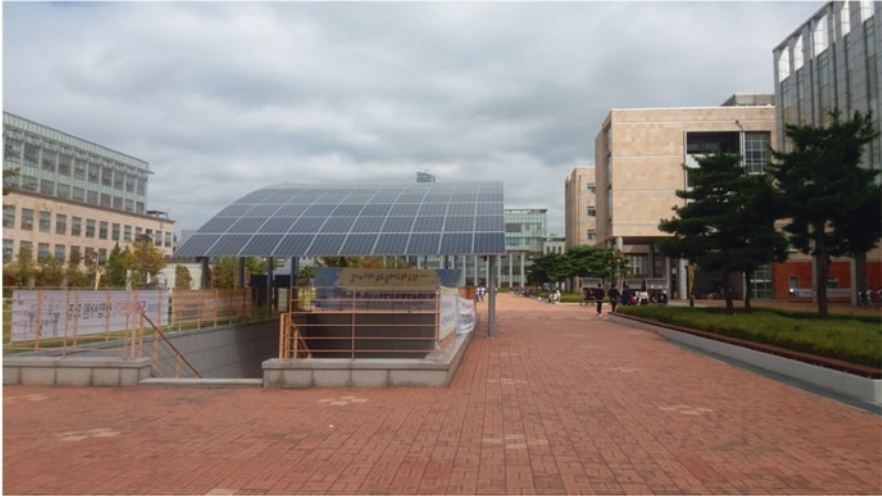
(a) Front view of a 180-solar PV array installed at Incheon National University green campus
