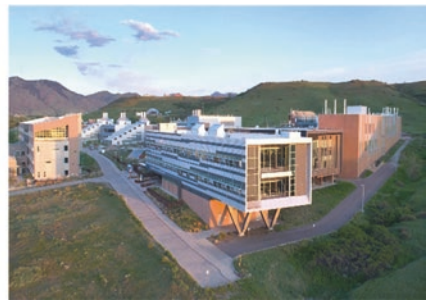
(b) The NREL buildings integrated with energy systems for a zero-energy target
