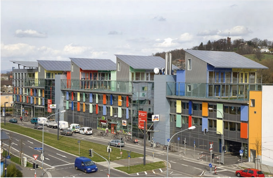
Fig. 48 The Sun Ship's retail, commercial, and residential integrated building. (Image credit and source: Andrewglaser, https://commons.m.wikimedia.org/wiki/File:SoSchiff_Ansicht.jpg#mw-jump-to-license )
