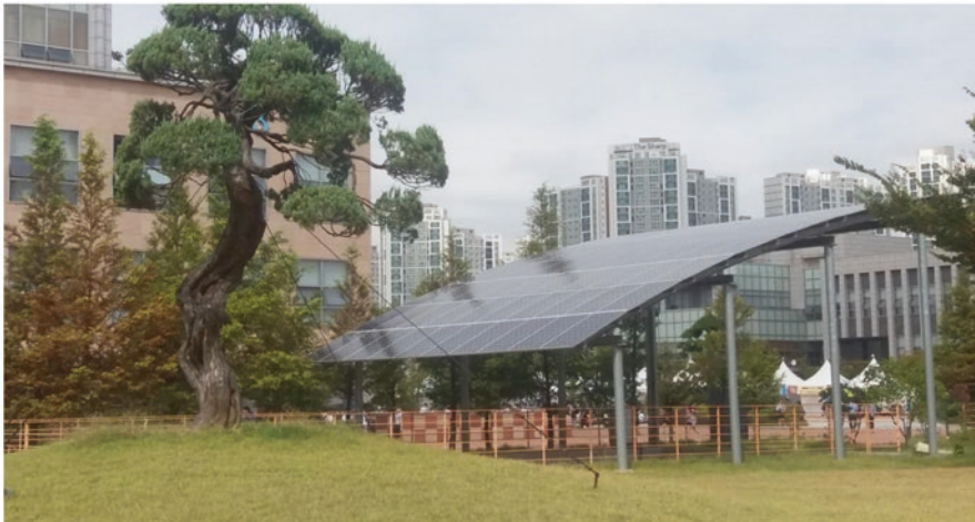
(b) View of a 180-solar PV plant installed at Incheon National University (INU) campus
