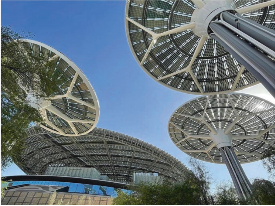
Fig. 5 A net-zero model (Solar Complex) Terra – The Sustainability Pavilion at Expo 2020 Dubai – by Grimshaw Global. (Image credit and source: Mohsen Aboulnaga & Amina El-Haggan)
