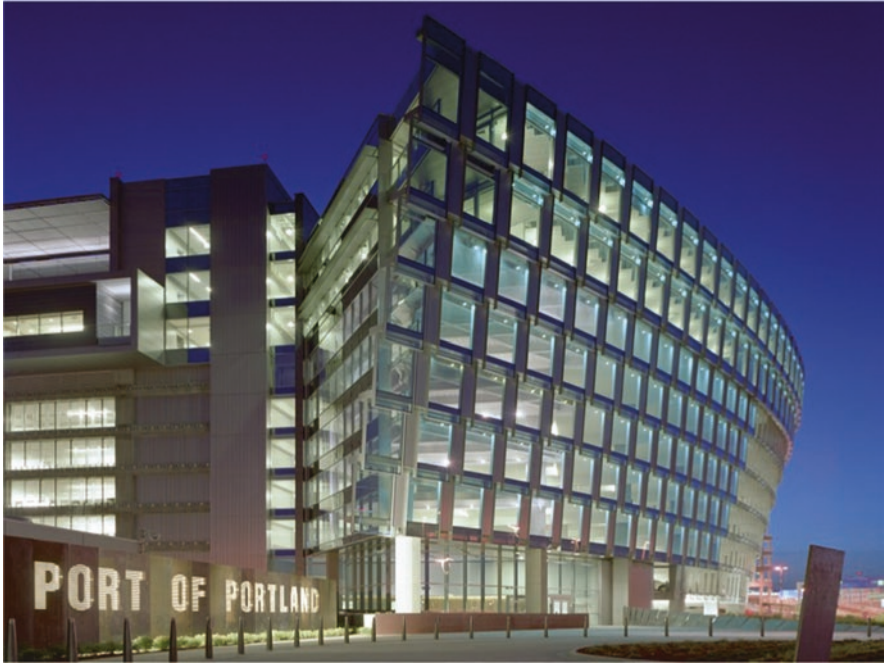
Fig. 62 Port of Portland Headquarters building. ( https://inhabitat.com/green-roofed-port-of-portland-headquarters-aims-for-leed-gold/ )
