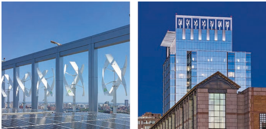
Fig. 8 Facade, photovoltaics, and wind turbine integration. Credit: FXCollaborative Architects LLP
