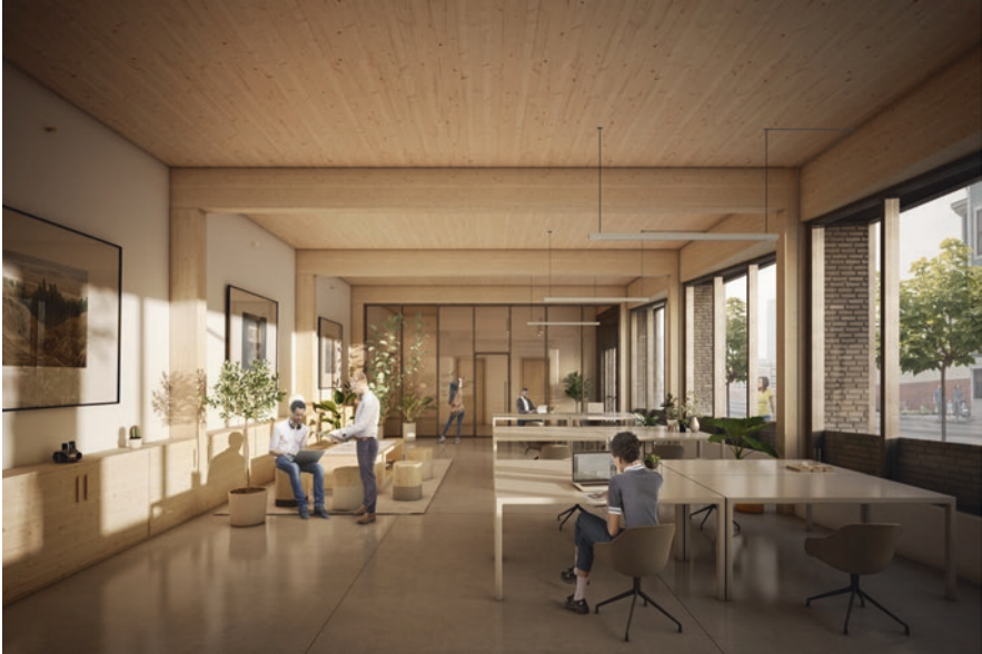
Fig. 17 CLT elements such as beams, columns, and ceilings can be seen from this render view. (Credit: Generate | Placetaylor)
