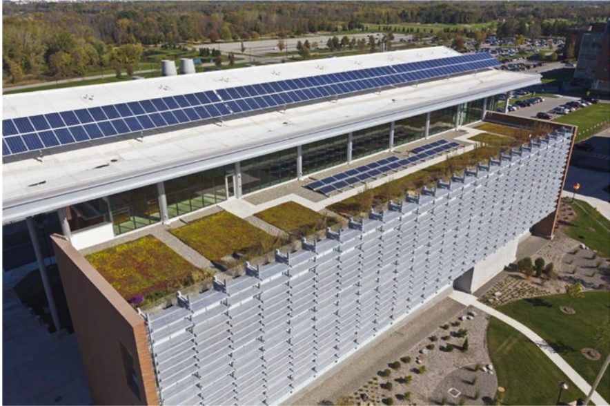
Fig. 28 Sun shading, PV systems, and green roof. Credit: Craig Shaw, Stratus Imaging
