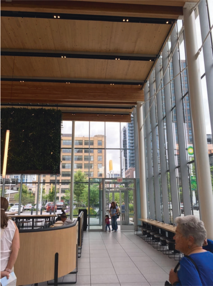
Fig. 46 The McDonald's Flagship was the first commercial building in Chicago to use timber framing as a primary structural element. (Credit: David Thaddeus)
