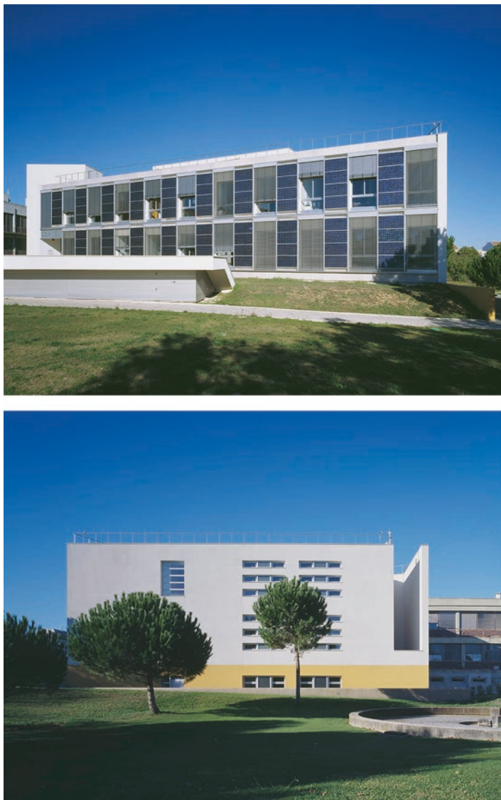
Fig. 20 The LNEC. South façade (above), East façade (below)
