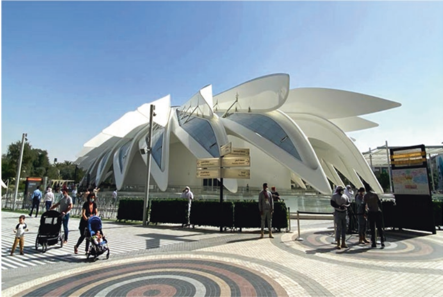
Fig. 16 The iconic UAE Pavilion with 28 floating wings integrating solar PV panels, EXPO 2020 Dubai. (Image credit and source: Mohsen Aboulnaga and Amina El-Haggan)
