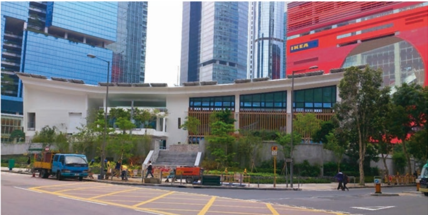
Fig. 24 Back view of the CIC Zero Carbon Building showing the solar PV panels on top of the roof. (Image credit and source: Ceeseven, https://commons.m.wikimedia.org/wiki/File:CIC_Zero_Carbon_Building.jpg )
