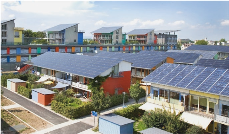
Fig. 45 Close-up of the Solar Settlements houses with PVs covering rooftops. (Image credit and source: Andrewglaser, https://commons.m.wikimedia.org/wiki/File:LuftSS.jpg#mw-jump-to-license )
