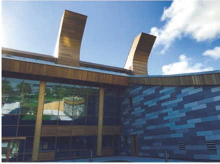
(a) Entrance to GSK Laboratory and its façades with efficient glass and cladding to save energy.
