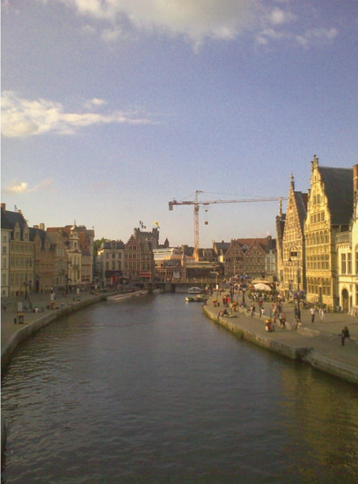
Fig. 3 Buildings in the medieval city of, in Belgium respond to climatic conditions and use less amount of energy due to locally sourced materials. (Image credit and source: Mohsen Aboulnaga)
