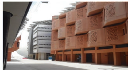
(b) Solar PV panels installed on buildings' rooftops
