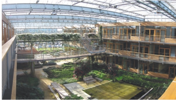
(a) Interior of Lumen greenhouse building illuminated naturally by daylight through glazed atrium.
