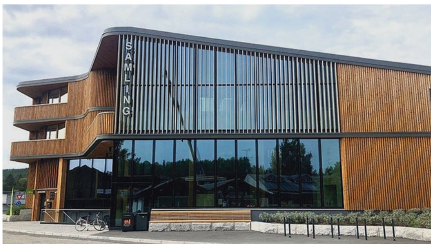
Fig. 57 The exterior of the Samling net-zero heating library in Nord Odal, Norway. (Image credit and source: Alek14, https://commons.wikimedia.org/wiki/File:Six-pane_application_in_Nord_Odal,_Norway.jpg )
