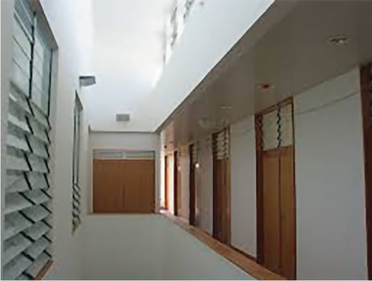
Fig. 21 The atrium: bioclimatic design for daylight and natural ventilation
