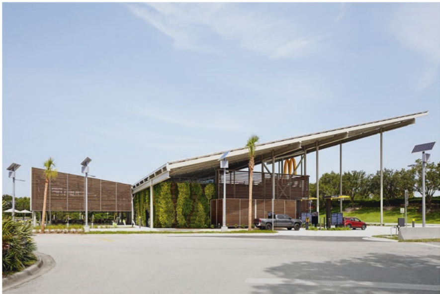
Fig. 36 A green wall equipped with a plant care system can be seen on the exterior of the building from the parking lot. (Credit: Kate Joyce Studios, McDonald's Flagship—Orlando, Ross Barney Architects, 2020)
