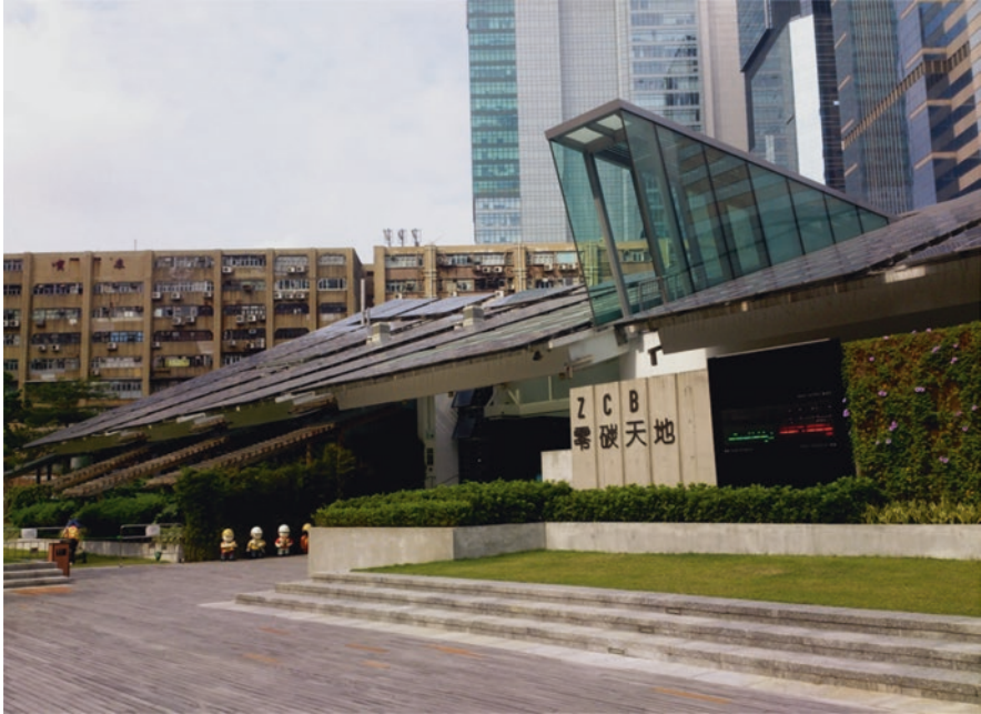
Fig. 25 The entrance of the CIC Zero Carbon Building showing the solar PV arrays. (Image credit and source: Ceeseven, https://commons.m.wikimedia.org/wiki/File:CIC_Zero_Carbon_Building.jpg )
