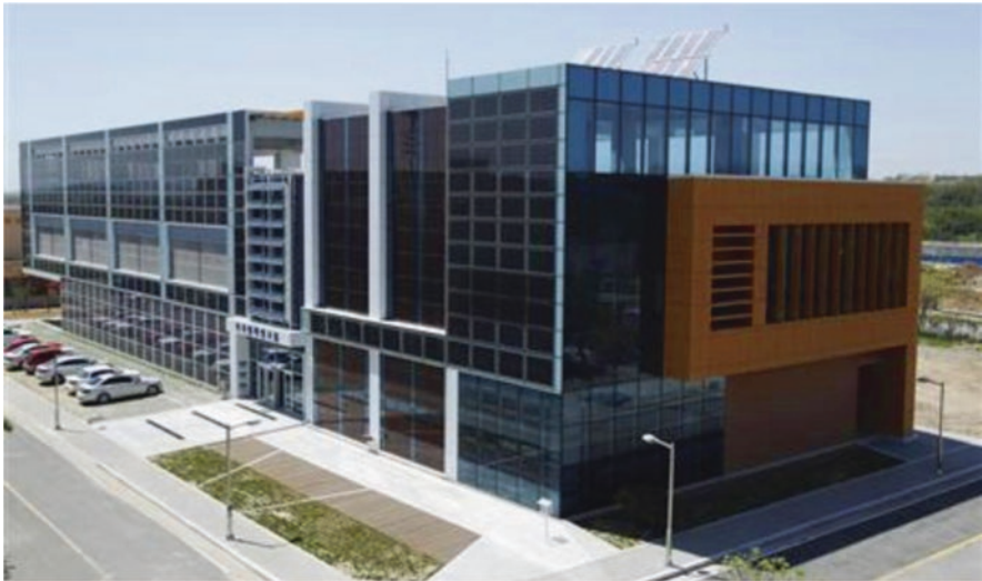
Fig. 27 Various types of solar PV panels installed on the façade of NEIR/CCRC building and solar collector arrays on rooftop. (Image credit and source: Truth Leem, Reuters https://www.reuters.com/articles/us-korea-green/south-korea-unveils-completely-eco-friendly-building-idINTRE74J1FE20110520 )
