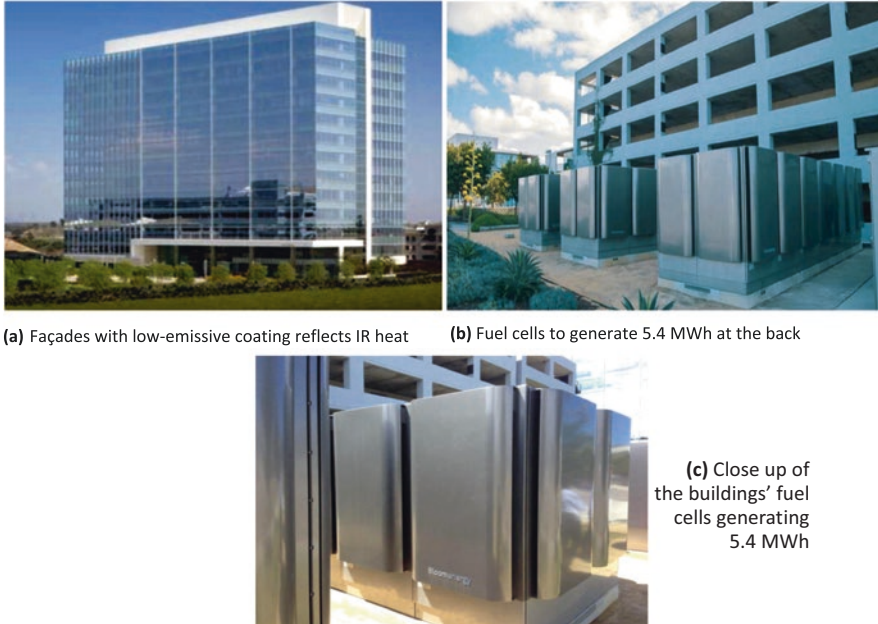
Fig. 55 The La Jolla Commons net-zero building in San Diego, CA, USA. (Source: (a–c) https://www.researchgate.net/publication/341264745_Net-Zero_Energy_Buildings_Principles_and_Applications ). (a) Façades with low-emissive coating reflects IR heat. (b) Fuel cells to generate 5.4 MWh at the back. (c) Close-up of the buildings' fuel cells generating 5.4 MWh
