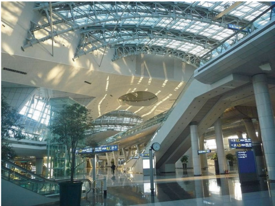
Fig. 30 Interior of Incheon-Seoul Airport Terminal, South Korea, a near-zero-energy building. (Image credit and source: Eliazar Parra Cardenas, https://commons.m.wikimedia.org/wiki/File:Incheon_airport.jpg )
