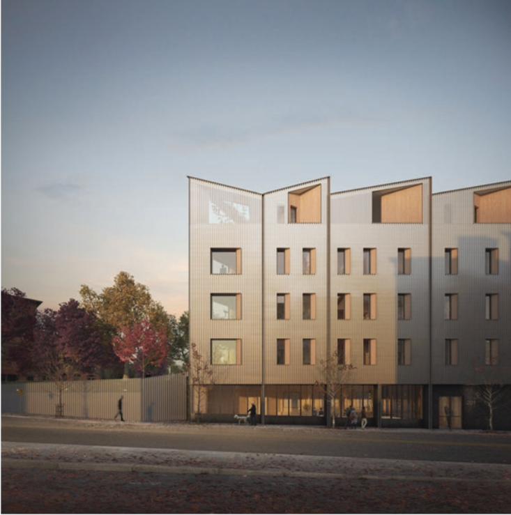
Fig. 18 Lightweight porous metal cladding will be used as the envelope of the building. (Credit: Generate | Placetailor)
