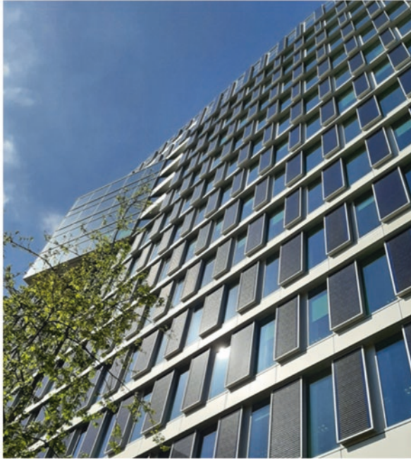
(a) A checkerboard of solar panels and windows to regulate heat and respond to weather conditions to minimise energy use
