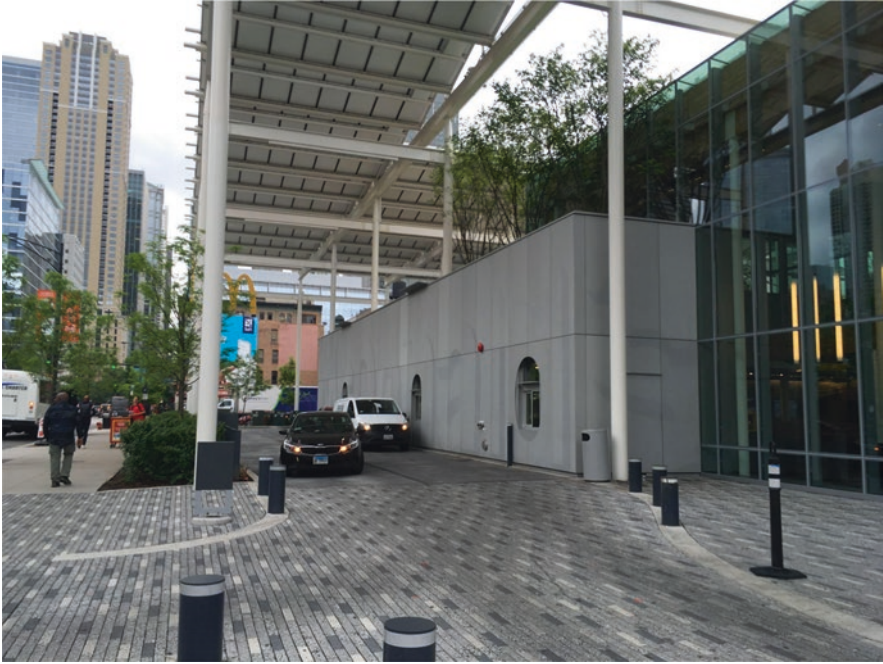
Fig. 48 The solar pergola hovers over the car lane providing shade and generating energy. (Credit: David Thaddeus)
