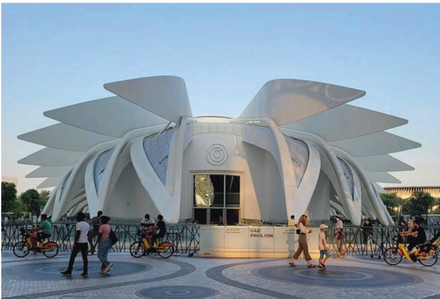
Fig. 17 The floating wings generate clean energy from renewable sources for the building energy annual consumption. (Image credit and source: Mohsen Aboulnaga and Amina El Haggan)
