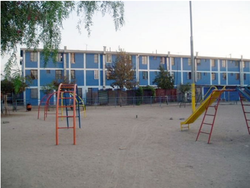
Photo 12.1 Remodeled children's playground together with painted facades in the CPTED el Caleuche project
