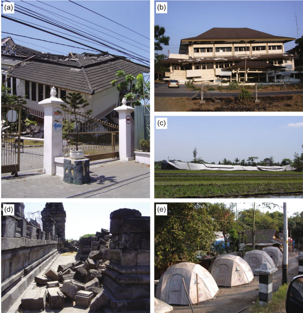
Fig. 1.16 Impact of the 6.4 Bantul earthquake south of Merapi on 27 May 2006. a-c Severe building damage in and around Yogyakarta. d Damage to Candi Prambanan. e Temporary shelters for earthquake victims near the village of Bantul. The earthquake caused more than 6,000
