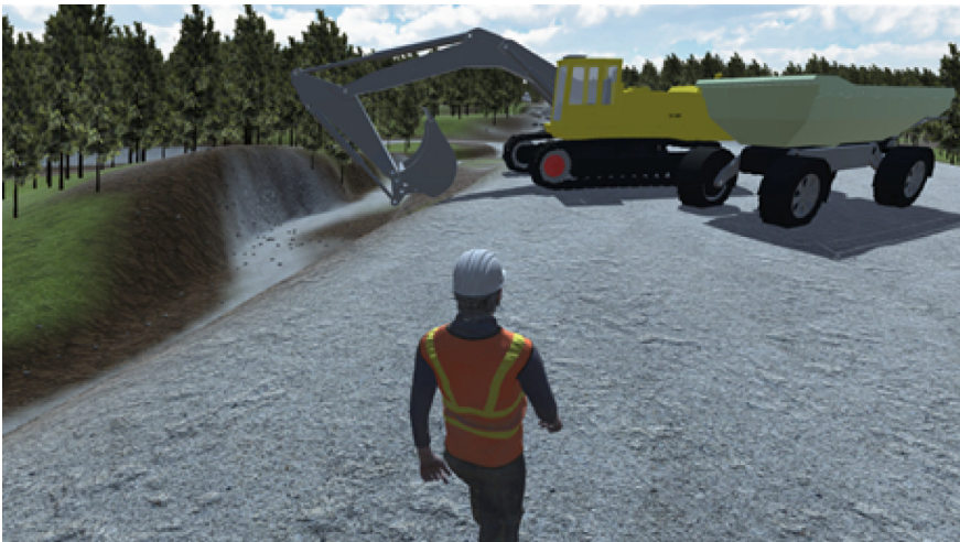
Fig. 5. The user can explore the site following a virtual operator showing the construction equipment and operations.
