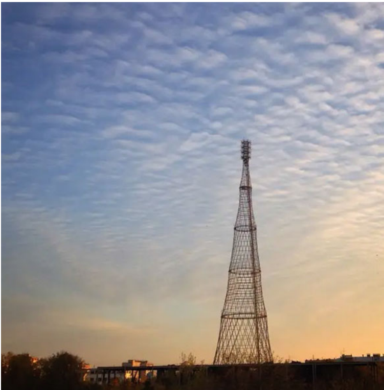
Fig. 1 The Shabolovka radio station in Moscow
