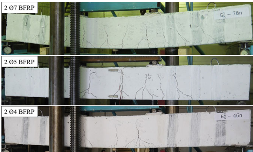
Fig. 18 Typical stages of crack development in beams of series 3, reinforced with two bars 2 Ø7 BFRP, 2 Ø5 BFRP and 2 Ø4 BFRP
