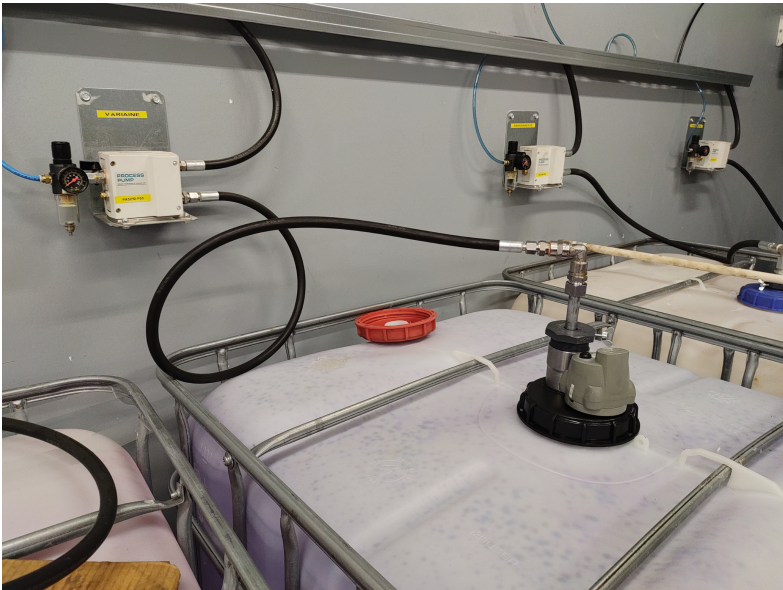
Fig. 2. The IoT sensor module installed in the cap of the marking colour container.
