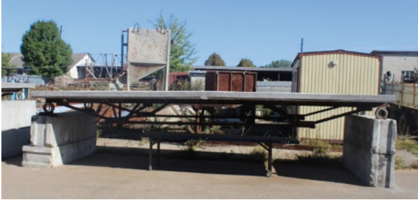
Fig. 5. General view of the experimental full-scale construction.
