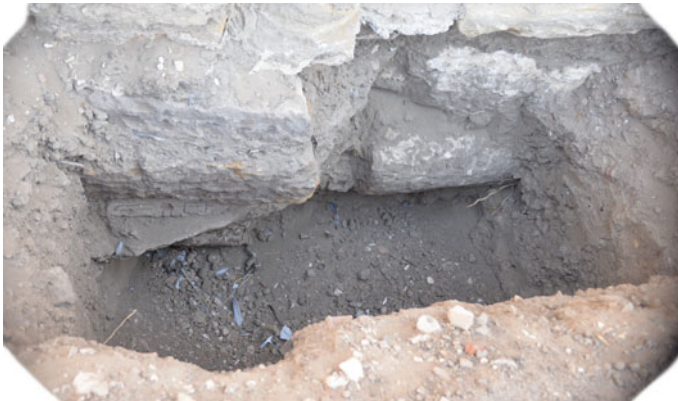
Fig. 10 Open pit showing shallow foundation of chapels walls
