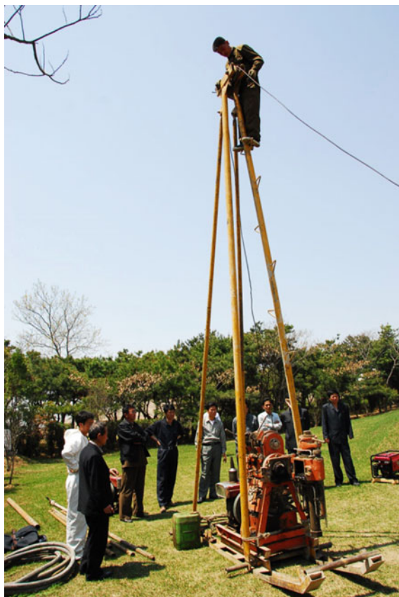
Fig. 5 The rotary/percussion machine in borehole S1
