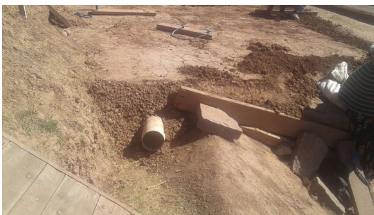
Fig. 17 Drainage pipe located in the back side of the gabion
