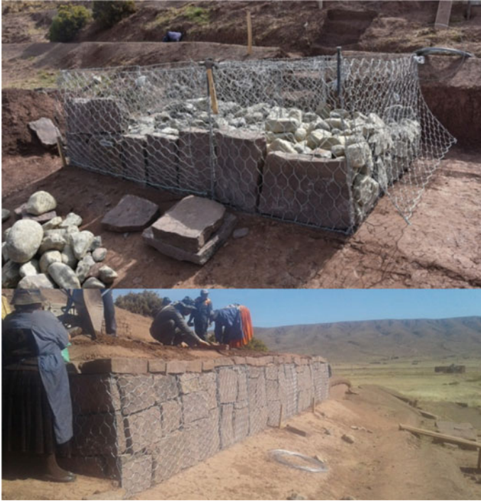
Fig. 22 Front view of the gabions adopted to reduce the visual impact
