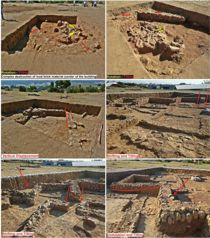
Fig. 12 Rotation, tilting, vertical displacement, shifting, undulation, uplift and complex destruction indications observed in the buildings located in the Ağılönü area
