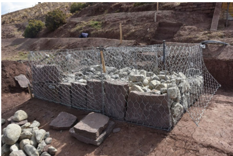
Fig. 16 Example of local stone (Arenisca) to be used for the external part of the gabions
