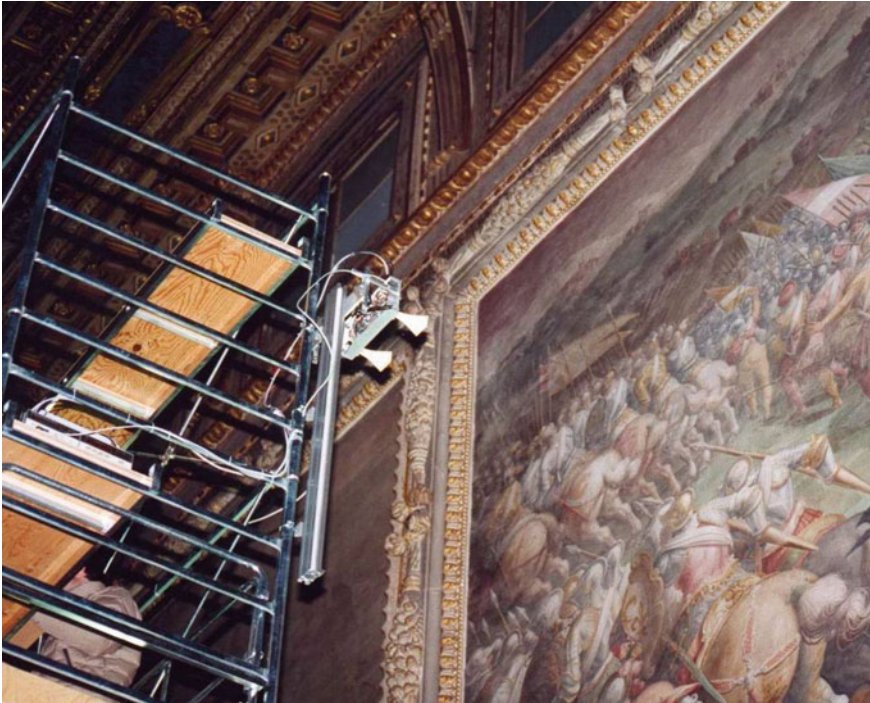
Fig. 7 No-contact high frequency GPR operating on the east wall of the Great Hall
