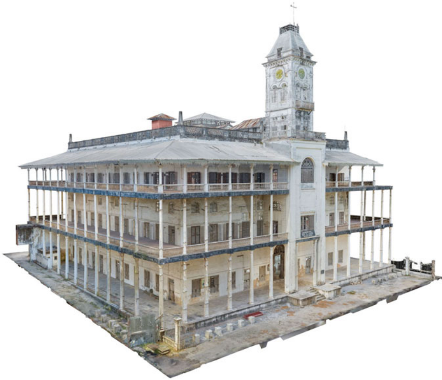
Fig. 4 House of Wonders, Stone Town Zanzibar. Decimated to 10 million surfaces or 0.2% of the originally acquired data for practical use
