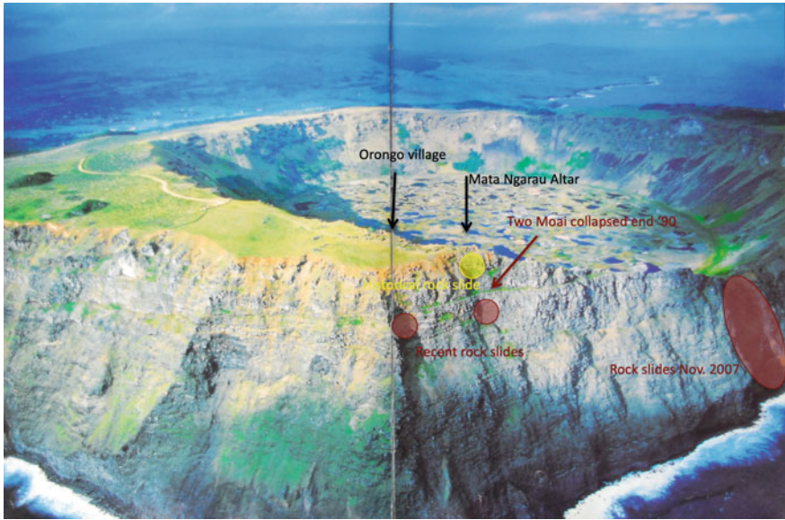
Fig. 5 Instability processes affecting the area immediately beneath the Orongo village
