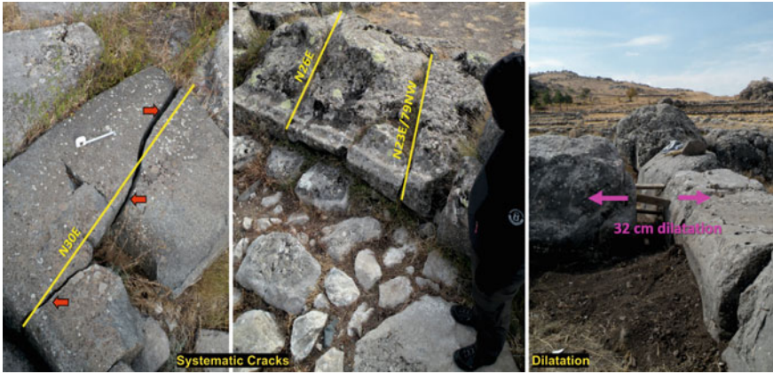
Fig. 24 Systematic cracks and dilatations on the Great Temple in the Lower City of Hattuša
