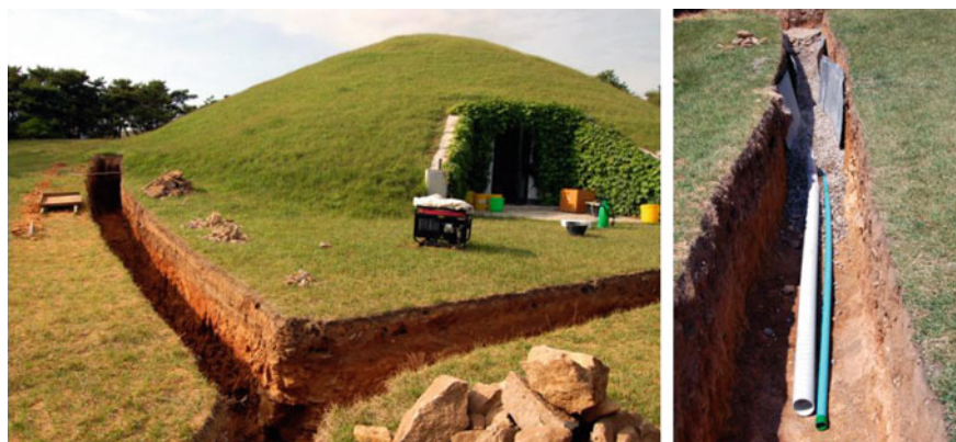
Fig. 19 Construction of the drainage trench
