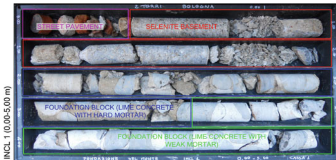
Fig. 4 Picture of cores extracted from the upper 5 m of one of the two inclined boreholes executed on the Asinelli foundation (INCL 1, dashed line on Section A-A, in Fig. 3) (modified from Marchi et al. (2019))
