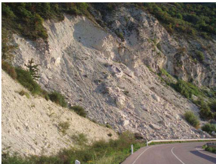
Fig. 1 Landslide, Paphos-Limassol Highway in Cyprus
