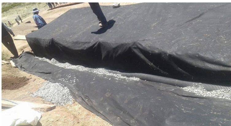
Fig. 18 Geotextile installation on the back side of the gabion
