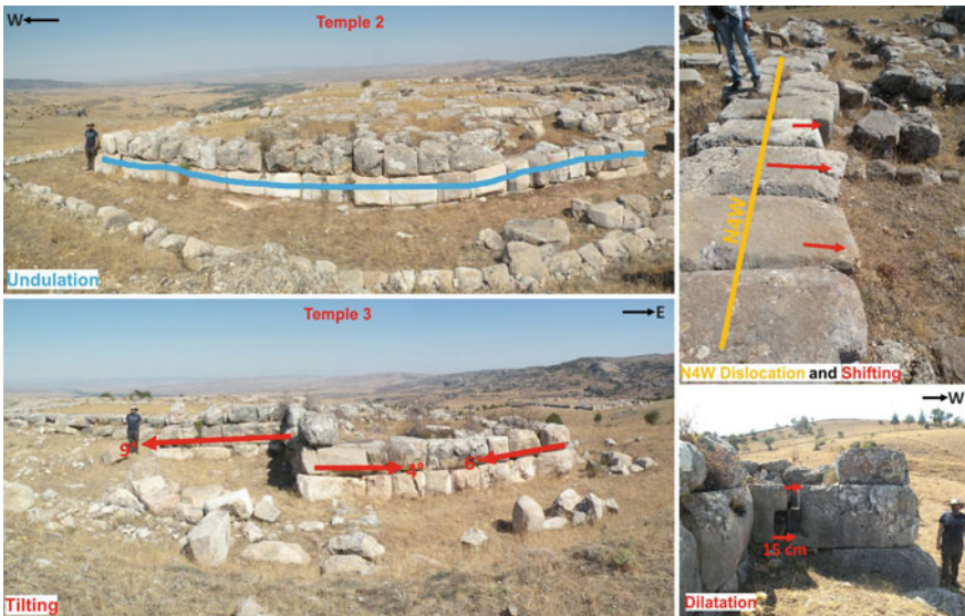
Fig. 18 Tilting, shifting, undulation, dilatation and dislocation type deformations in The Temple's district
