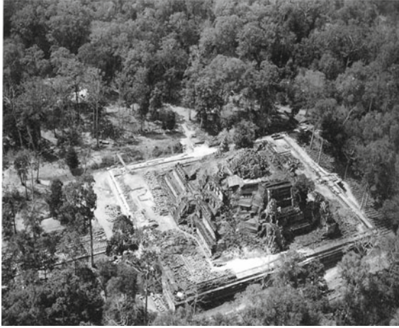
Fig. 20 Slope failure of the Baphuon in 1943 (1963, EFEO) (Pascal 2016)
