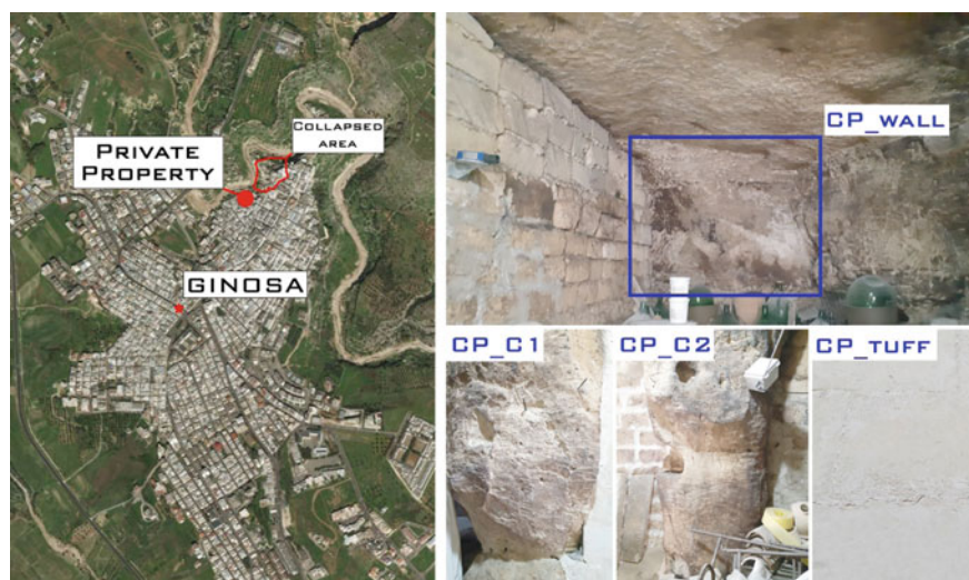
Fig. 4 Location of the private cavity in Ginosa and collapsed area
