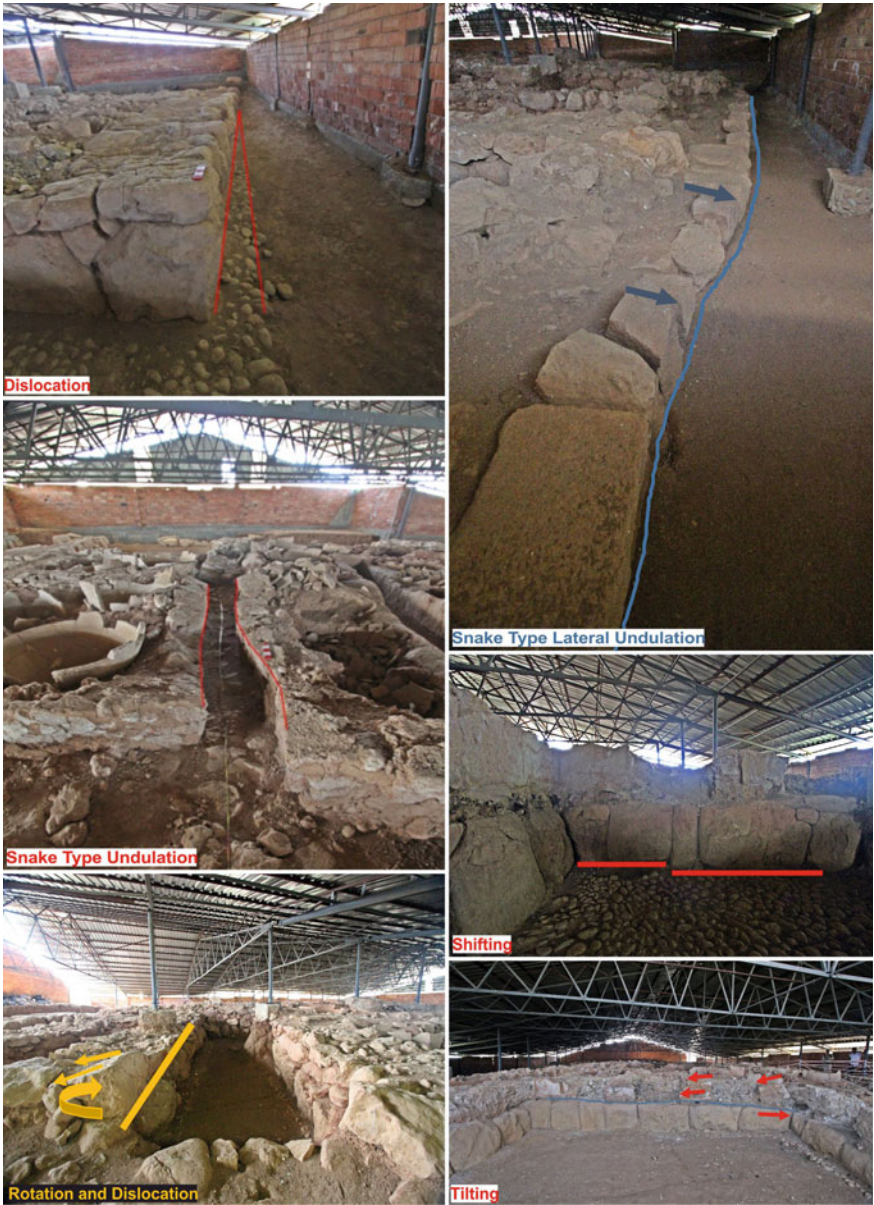
Fig. 8 Archaeo-seismologic deformational structures on the building “B”, tilting, shifting, snake-type lateral undulations, dislocations and rotations
