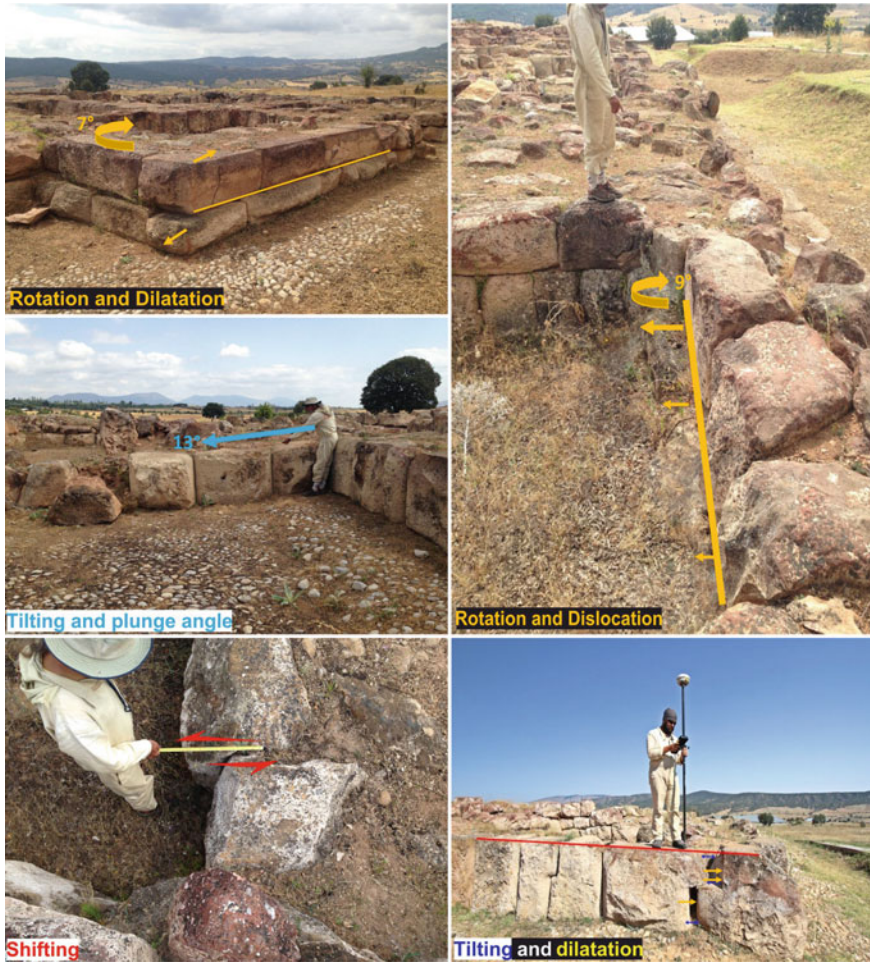
Fig. 6 Seismo-gravitational deformation structures on the building “A”, a some rotation, dislocation, tilting, dilatation and antiformal type and b synform, shifting type deformations
