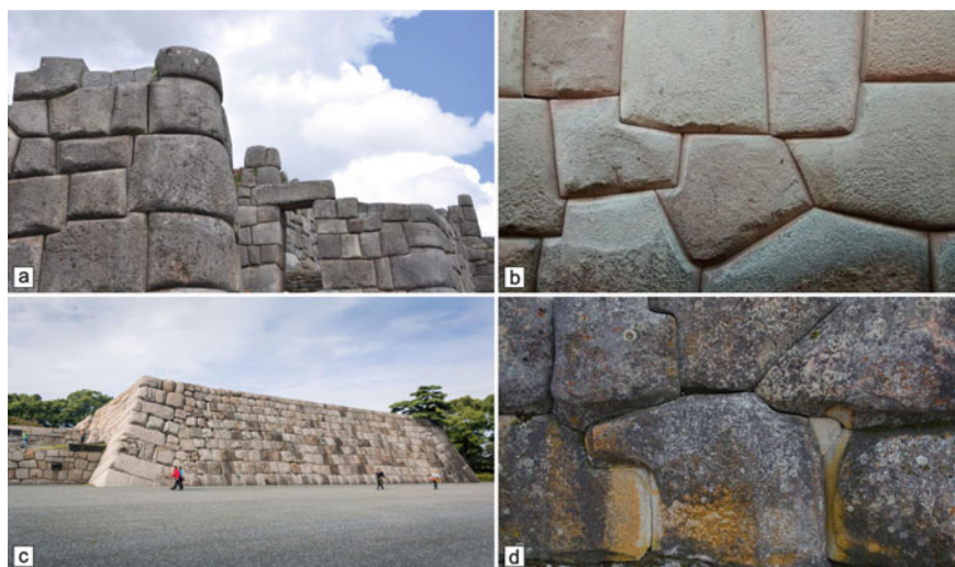
Fig. 3 Seismically isolated wall examples. Inca walls from a Sacsayhuamán b Cusco ( https://paleoseismicity.org/active-faults-around-cusco-peru-field-work-on-paleoseismology-and-archaeology-for-project-cusco-pata/ ), c Tokyo castle wall from Medieval Age ( https://www.worktravelshoot.com/2018/11/Walkthrough-guide-tokyo-imperial-palace-east-gardens.html ), and d Hittite wall from Alacahöyük ( https://mapio.net/pic/p-12656965/ )
