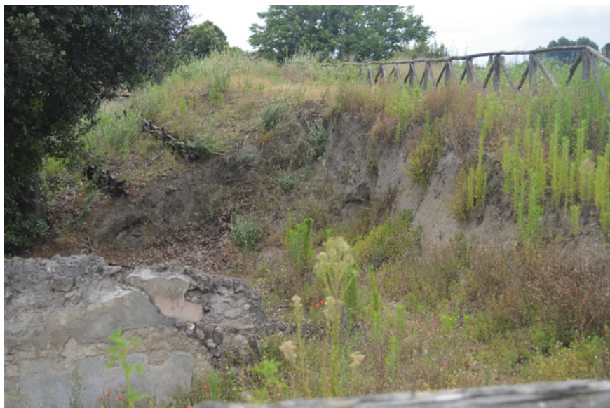
Fig. 4 Instability process affecting small portion of the unexcavated slope in the northern sector (Regio V)
