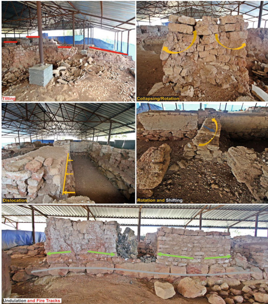
Fig. 10 Deformational structures and significant fire tracks on the building “D”
