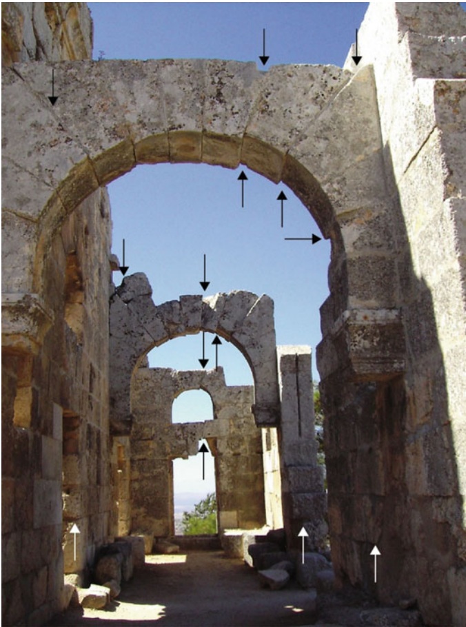
Fig. 6 Earthquake damage on arches of the Qalaât Samaan (Saint Simeon) Basilica. Earthquake damage (arrows) consists in displaced arches with shifted keystones, waved walls, turned columns and horizontal shifting of building stones. Written accounts and archeological investigations correlate the main earlier damage to the 29 May 526 earthquake (M 6.5, Table 1)
