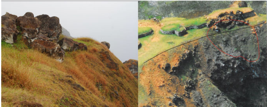
Fig. 6 The area below Mata Ngarua were a shallow landslide on weathered lava/debris/vegetation, possibly occurred in the past
