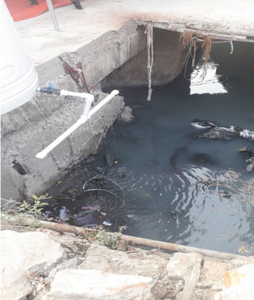
Fig. 8 Application of eco-enzyme at sewage drain (Mukeri ganj Nala, Azamgarh)
