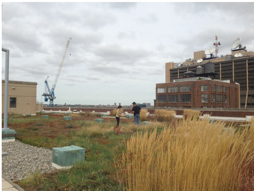
Fig. 10.3 United States Postal Service Morgan Center Processing Plant Sedum sp. green roof showing considerable contamination of non- Sedum grasses
