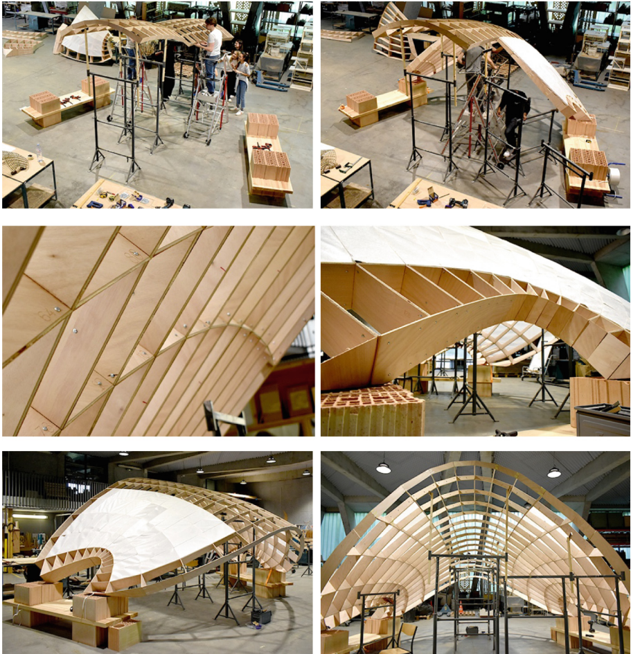
Fig. 21. The assembling of the partitions into the fully assembled model.
