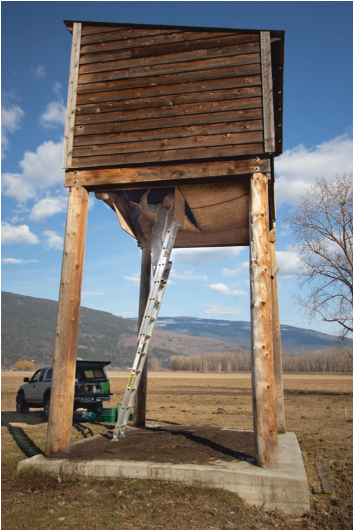
Fig. 6.3 A 'bat condo', an elevated structure built with many chambers inside to house thousands of bats. (Photo by Jared Hobbs)
