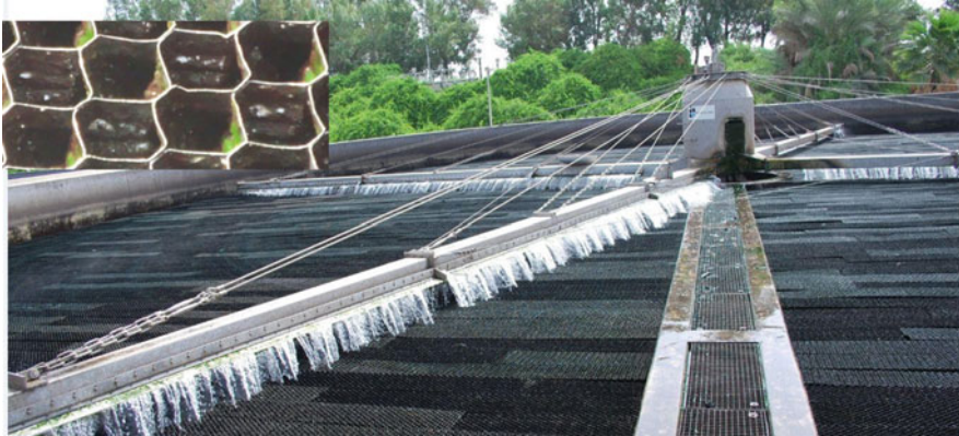
Fig. 6 The random media being used in the trickling filters
