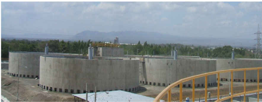
Fig. 2 Wastewater treatment plant of Managua: 6 trickling filters
