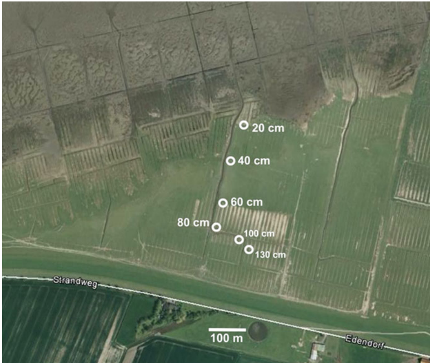
Fig. 4.10 Research area at the foreland of Friedrichskoog. White circles indicate the locations of sampling stations (Image: Google Earth; geographical coordinates: 54°02′35″ N, 8°52′48″ E)
