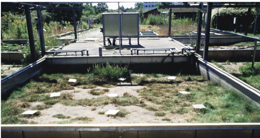
Fig. 20.1 One of the three tide simulation basins with the control panel in the centre for flooding regulation. The salt water tank is located under the panel
