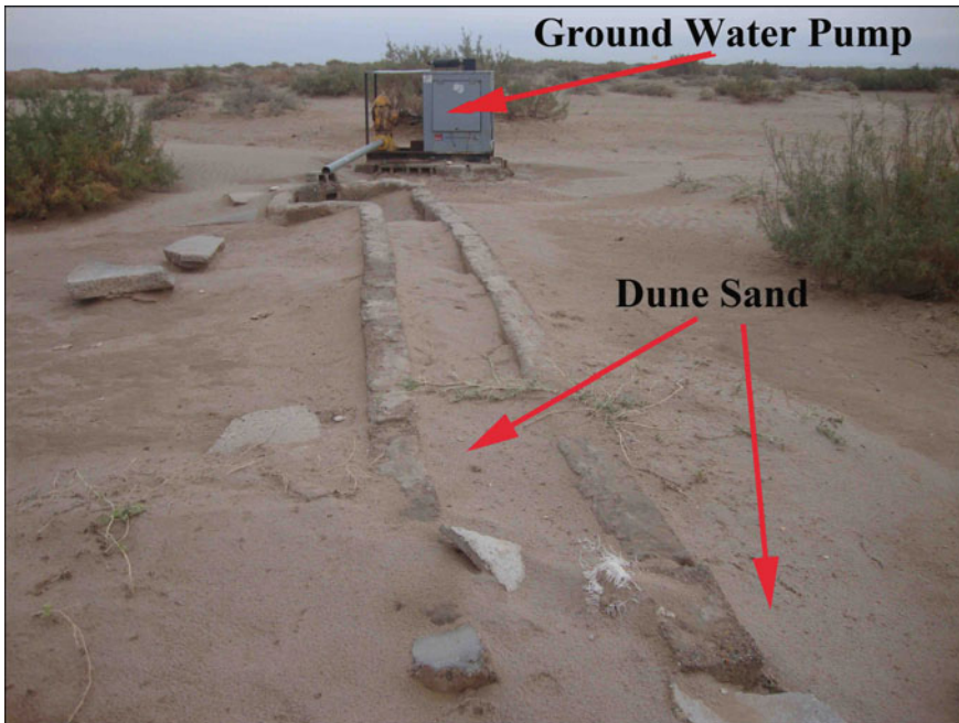
Fig. 23 Artificial channel for pumping ground water occupied by dune sands in Missan Governorate
