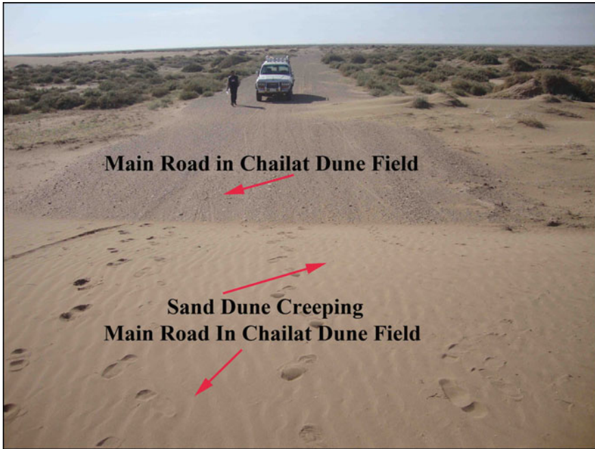
Fig. 7 Main road closed by migration of sand dunes in Missan Governorate, Middle Chailat dune field
