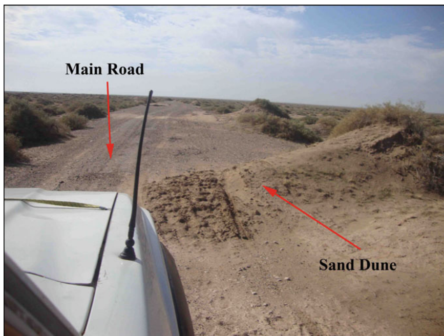
Fig. 8 Road closed by migration of sand dunes in Missan Governorate, Middle Chailat dune field
