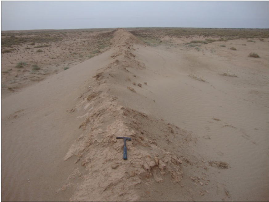
Fig. 20 Dune sand creeping on the soil bar for stabilizing sand dunes migration (the bar traps the dune sands) in Middle Chailat dune field. Missan Governorate
