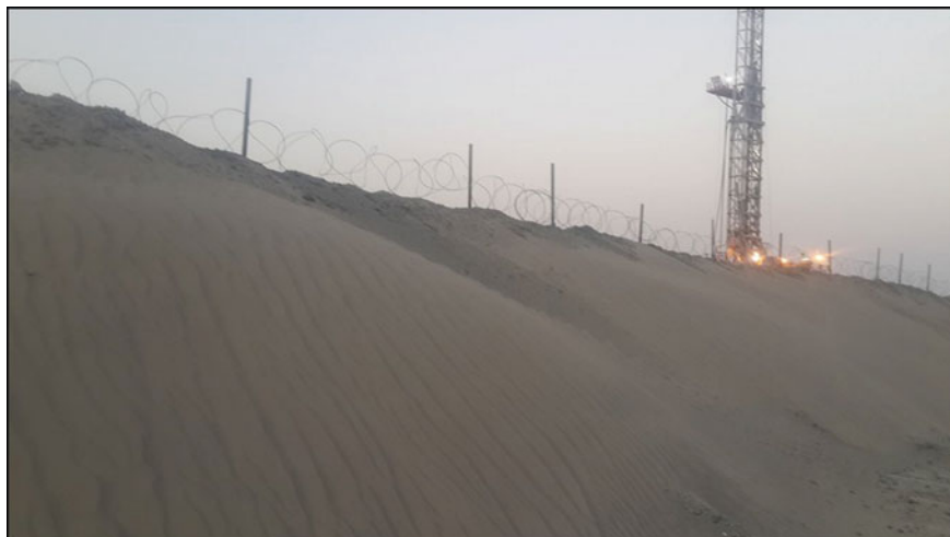
Fig. 18 Sand dunes creeping over fences of oil insulation in Thi-Qar Governorate
