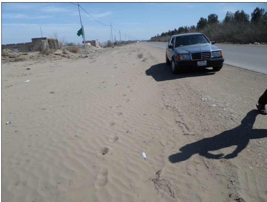
Fig. 10 Sand dunes deposited on the side of the road in Thi-Qar Governorate
