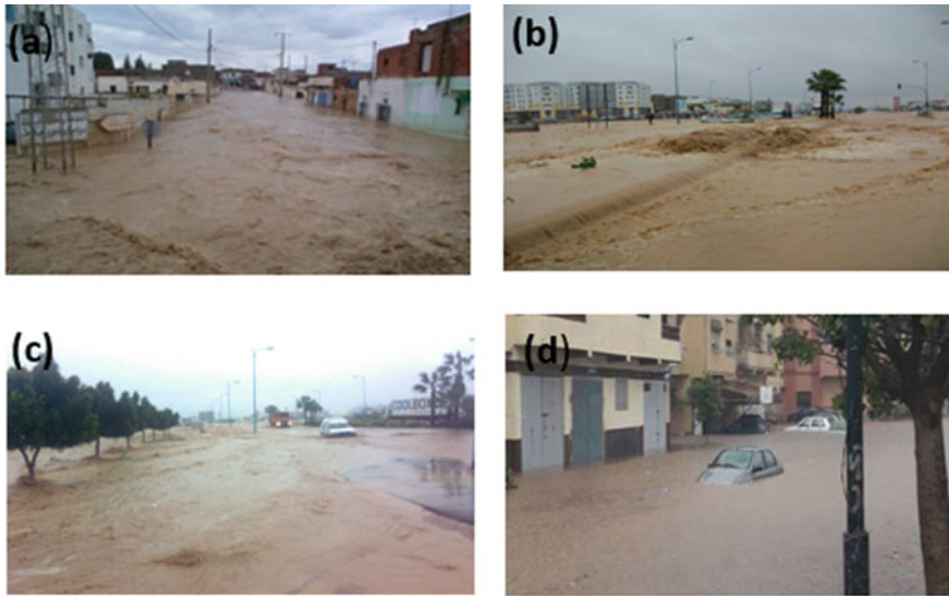
Fig. 16.4 Photos showing infrastructure damage to urban areas during the 2010 and November 2014 floods
