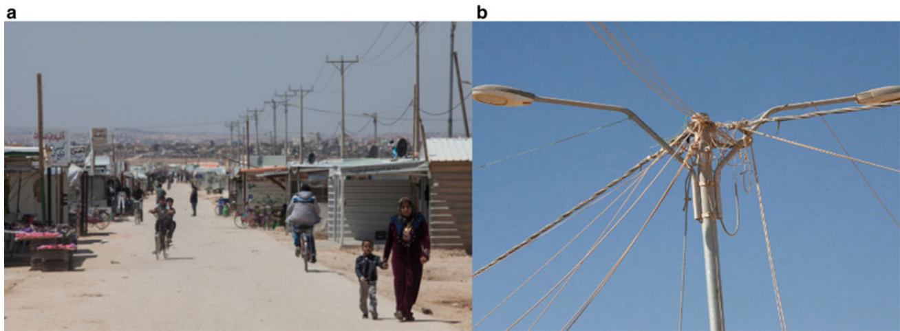
Fig. 3 a Electricity wires in Zaatari camp UNHCR (2017). b Illegal wireless connection. From Ledwith (2014, p. 33)
