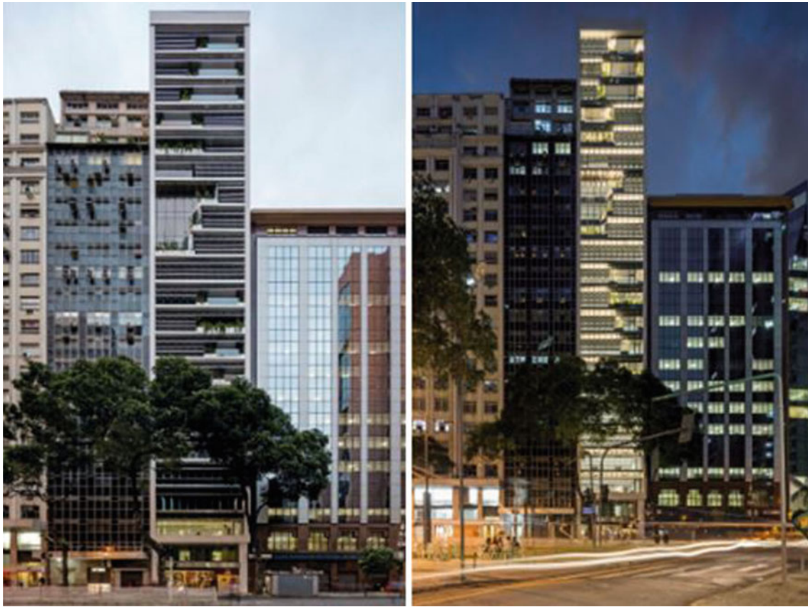
Fig. 16 RB12 bioclimatic diamond façade after building renovation at daylight and night (Finotti, 2016)
