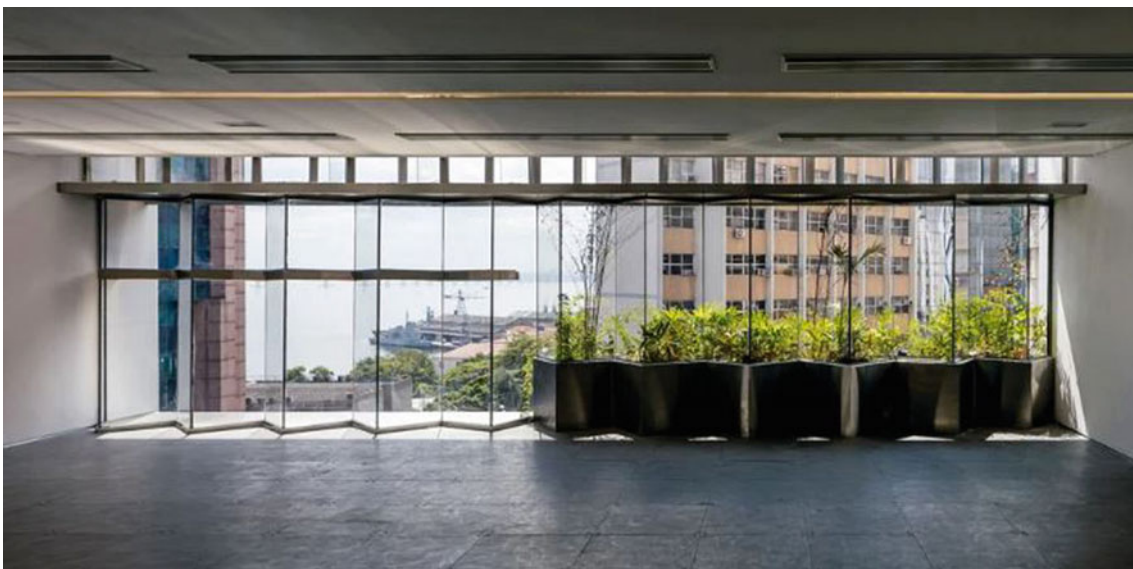
Fig. 17 RB12 bioclimatic winding facade from inside (Finotti, 2016)
