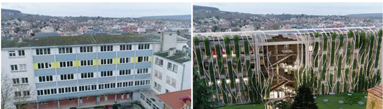
Fig. 18 CDER building before and after renovation design (OuyOut, 2019)
