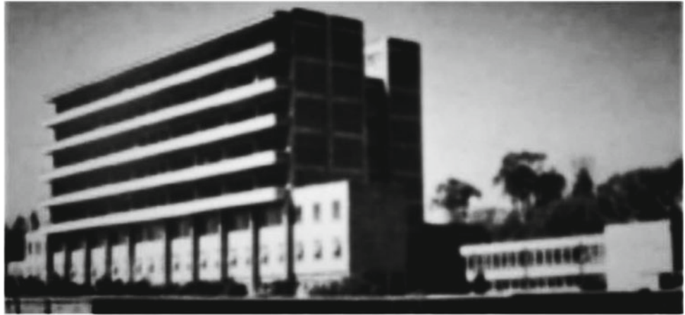
Fig. 10 Manuel Gea González Hospital original façade (Bitencourt & Monza, 2017)
