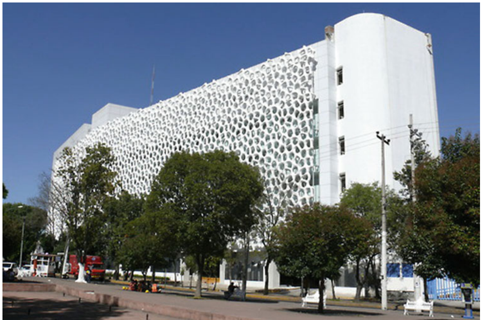
Fig. 11 Manuel Gea González Hospital renovation façade (Embellishments, 2014)
