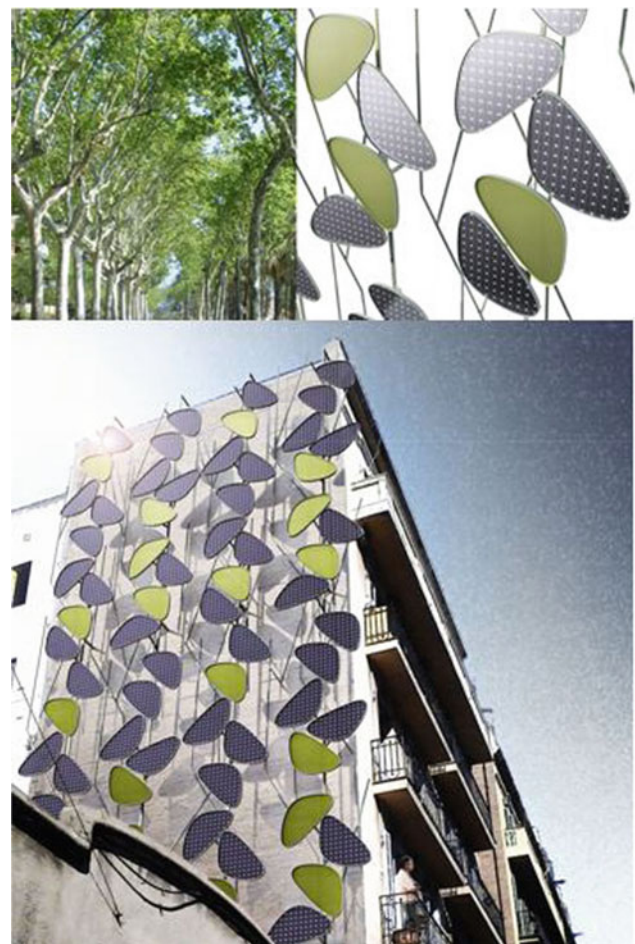
Fig. 14 Series of leaves shape panels applied on an old building in Barcelona (Samper & Juncadella, 2014)
