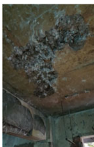
Fig. 3 Leaching of calcium carbide from slabs during water spray
