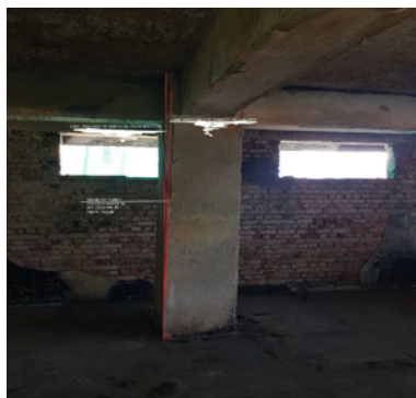
Fig. 4 Angular displacement on column
