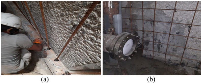
Fig. 8 a Fixing of rebars using anchor grout, b Reinforcement jacketing (typical)
