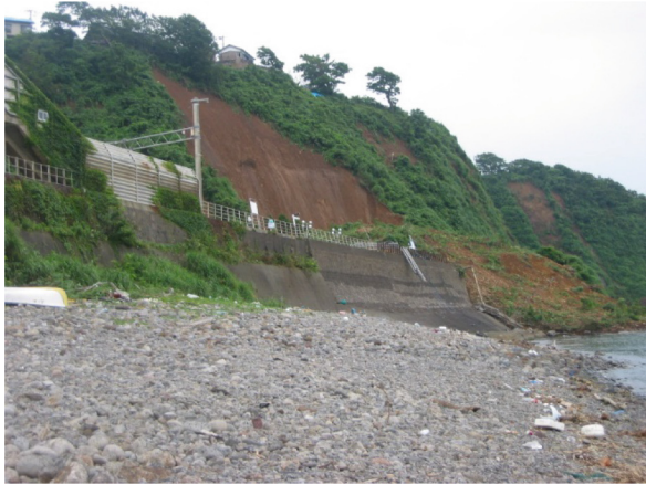
Fig. 2. Omigawa landslide triggered by the 2007 Chuetsu Oki earthquake, Japan. The landslide mass was formed in weathered sandstone on a steep slope of 55–60°.
