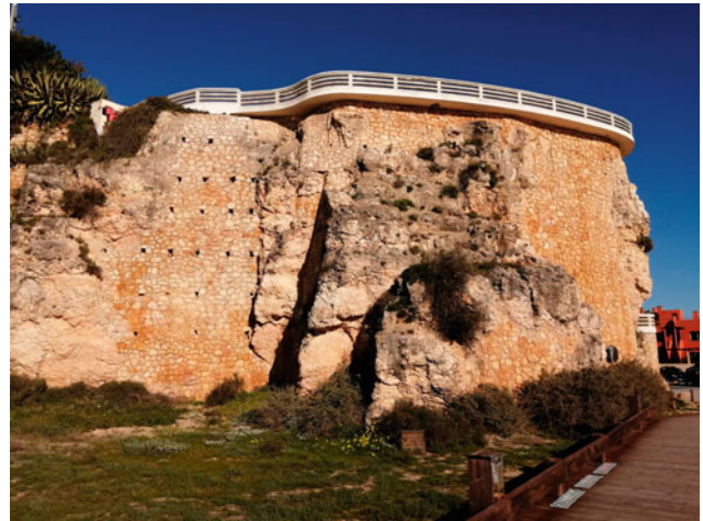
Fig. 4 The artificial cliff as it is in present day. It is in an advanced state of erosion. Photograph taken by the author in August 2021
