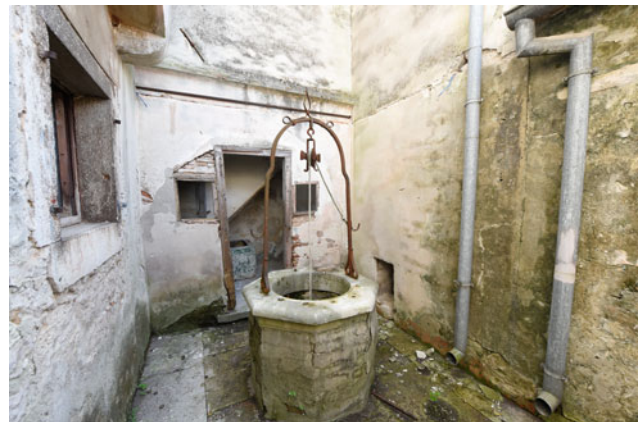
Fig. 10 Internal courtyard of the two houses before renovation. Credits Spirito Santo Palazzo Storico
