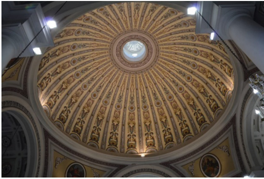
Fig. 8. Internal view of the dome.
