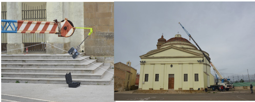
Fig. 3. TLS survey of the roof
