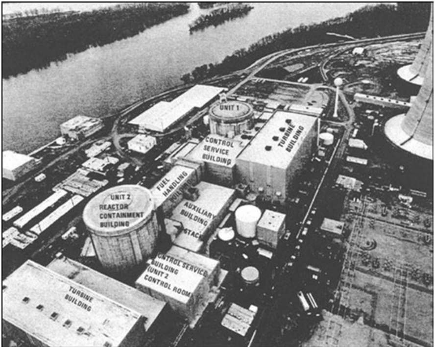
Photo 3.2 Unit-2 is in the foreground. The photograph is taken from one of the cooling towers of unit-2
