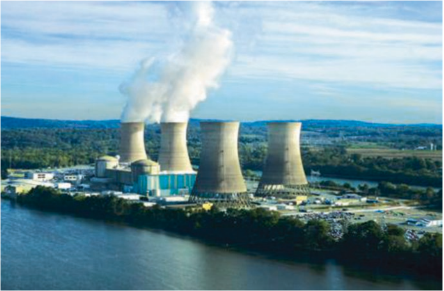
Photo 3.1 The Three Mile Island plant is located on an island in the Susquehanna River, 10 miles from the city of Harrisburg. The No. 2 reactor is the building with the rounded dome that is located closest to the two non-functional cooling towers. Those in operation produce steam cloud
