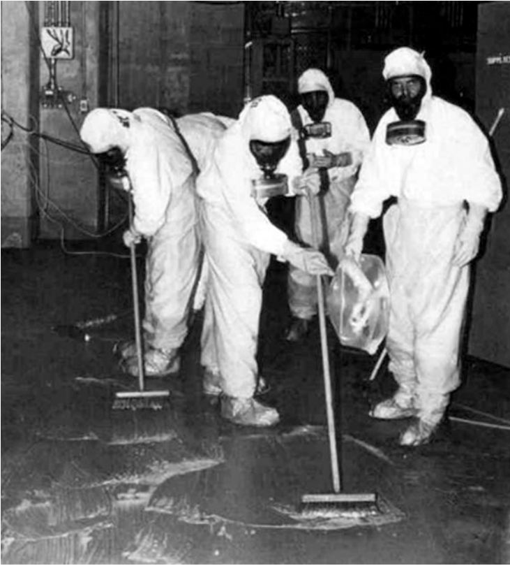
Photo 3.6 Cleaning the floor for decontamination
